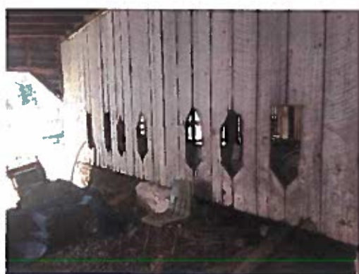
Photo L. Partition wall between central bay and 'right' bay. Ledger board visible at top. The wall has been painted, suggesting it may have been an exterior wall prior to the construction of the 'right' bay. Altered to create feed stalls.
