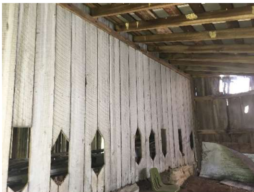
Photo K. Partition wall between central bay and 'right' bay. Ledger board visible at top. The wall has been painted, suggesting it may have been an exterior wall prior to the construction of the 'right' bay. Altered to create feed stalls.
