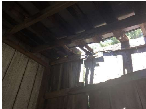
Photo F. Missing roof panels at rear wall.
