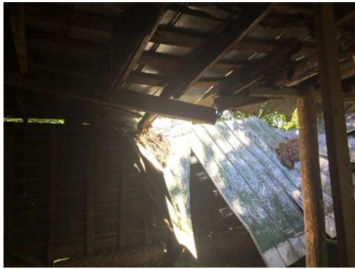
Photo I. Collapsed roof and end wall, and structural damage.
