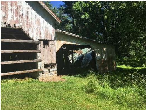
Photo C. 'Right' bay, with collapsed roof visible through opening.
