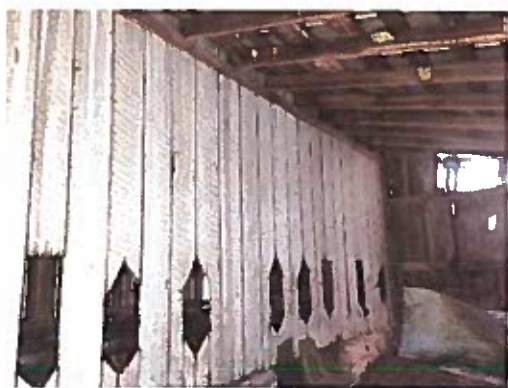
Photo K. Partition wall between central bay and 'right' bay. Ledger board visible at top. The wall has been painted, suggesting it may have been an exterior wall prior to the construction of the 'right' bay. Altered to create feed stalls.
