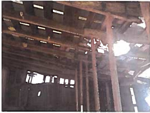
Photo G. Structural damage (broken roof rafters) and roof failure.
