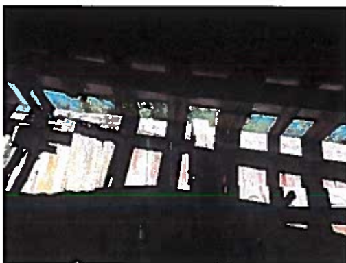
Photo E. Missing roof panels at rear wall
