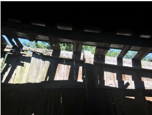
Photo E. Missing roof panels at rear wall
