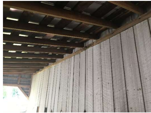
Photo J. Ledger board supporting roof rafters, at top.
