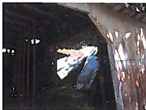
Photo D. Collapsed roof and end wall, visible through door. Note corrugated metal siding.
