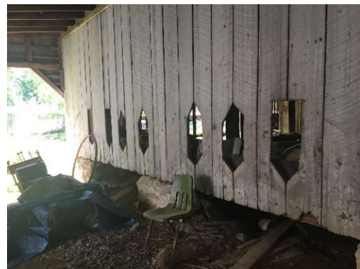
Photo L. Partition wall between central bay and 'right' bay. Ledger board visible at top. The wall has been painted, suggesting it may have been an exterior wall prior to the construction of the 'right' bay. Altered to create feed stalls.
