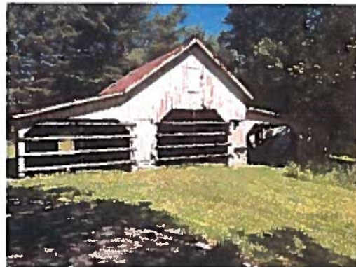
Photo B. Corncrib, showing the central and 'left' bays (to remain), and the partially collapsed 'right' bay. Note: Roofs of 'central' and left bays engage; the 'right' bay roof is disengaged.
