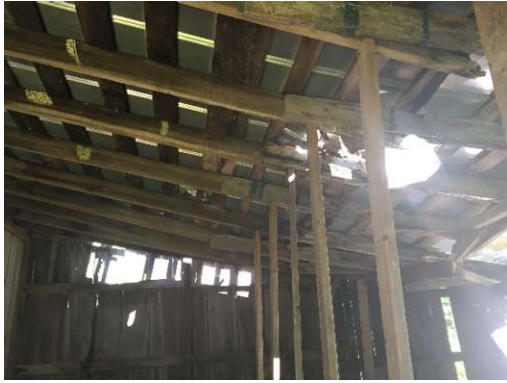
Photo G. Structural damage (broken roof rafters) and roof failure.
