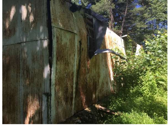
Photo N: Side elevation of 'right' bay, showing damaged wall.
