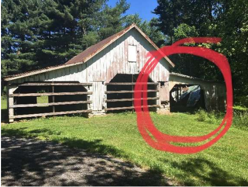
Photo A. Corncrib, showing the central and 'left' bays (to remain), and the partially collapsed, likely more recently constructed, 'right' bay (circled).
