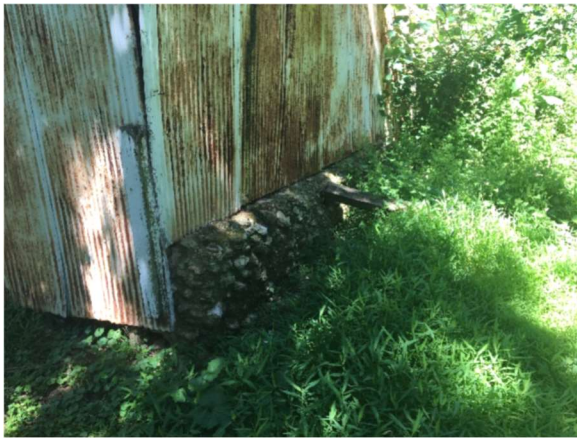
Photo O: Side elevation of 'right' bay, showing stone footer. Note difference in materials from 'central' bay pier.
