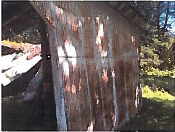
Photo M: Front elevation of 'right' bay. Note corrugated metal siding.
