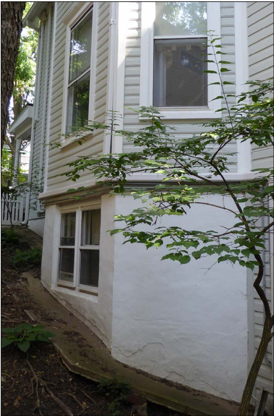
SOUTH-WEST SIDE: REPLACE EXISTING PAIR OF DOUBLE HUNG (NOT ORIGINAL TO THE HISTORIC HOUSE) WITH PAIR OF CASEMENTS FOR EGRESS
