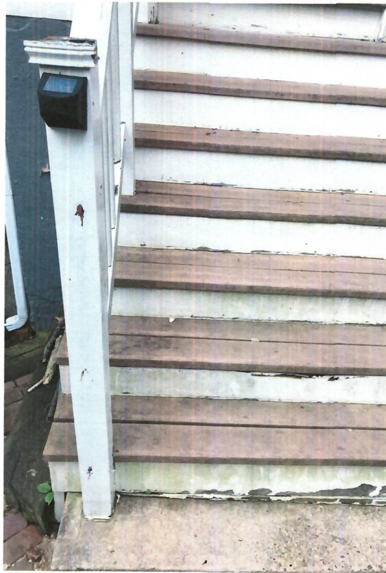
close-up to show composite material on steps - would be replaced with wood.
