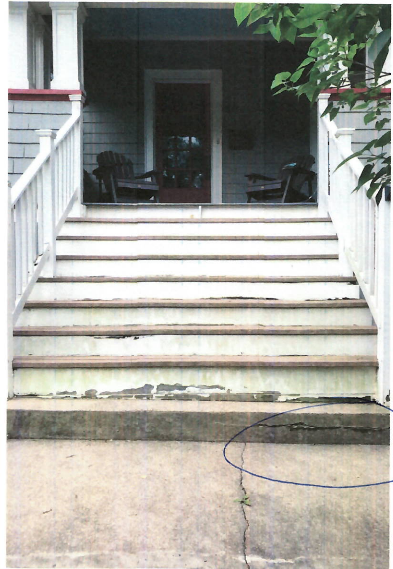
overview of current existing steps - steps would come out further to correct rise and run issues and cover bottom concrete step
