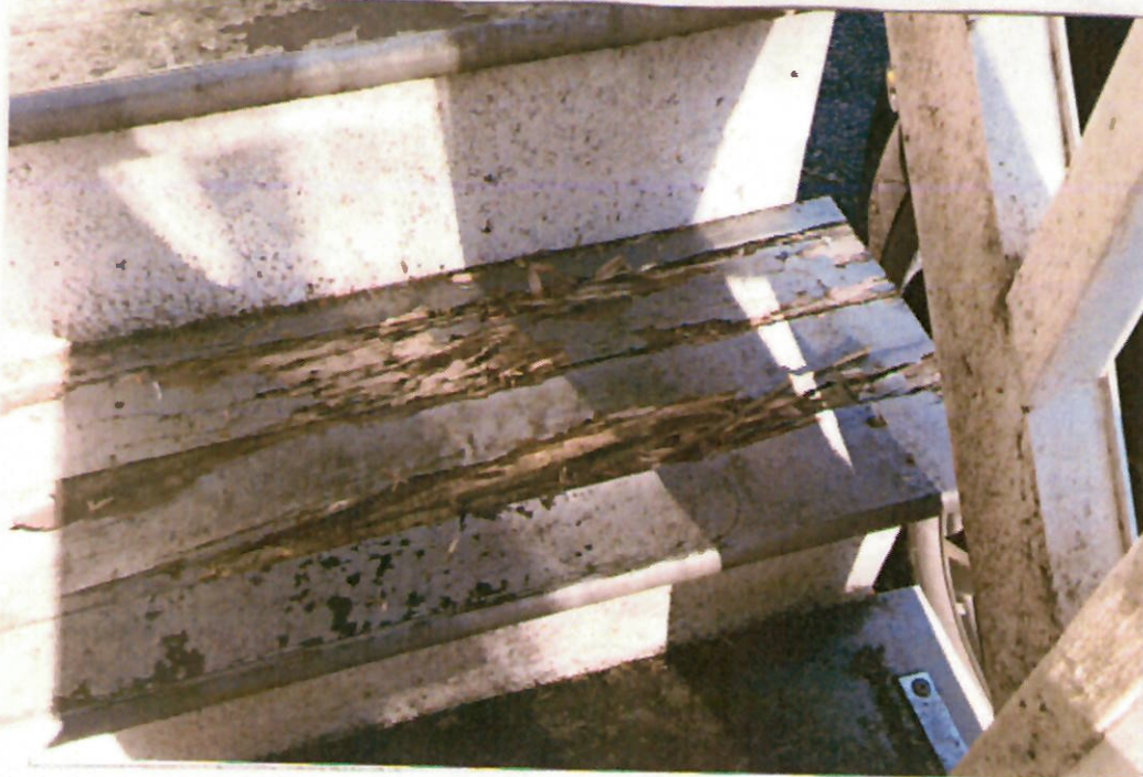
Detail: SIDE PORCH BROKEN/ROTTING STEPS
