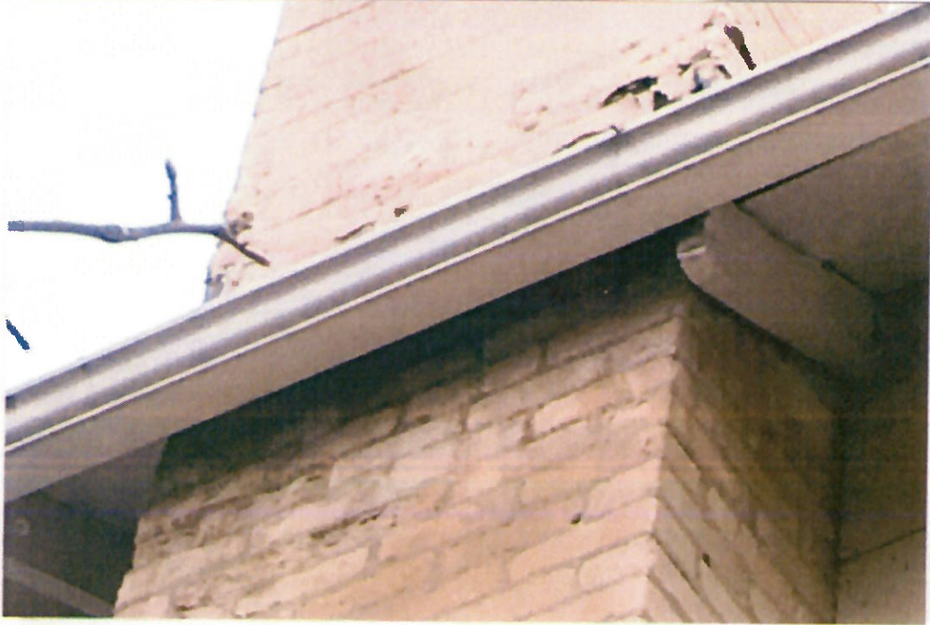
Detail: CHIMNEY DETERIORATING, BROKEN EAVE
