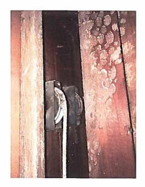
Photo J. Detail, pulleys from double-hung window
