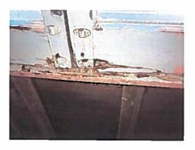
Photo F. Casement window, interior, showing hardware and damage
