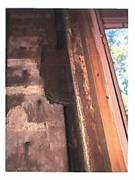
Photo B. Detail of 'strap pulley' cassette, set into four by four stud
