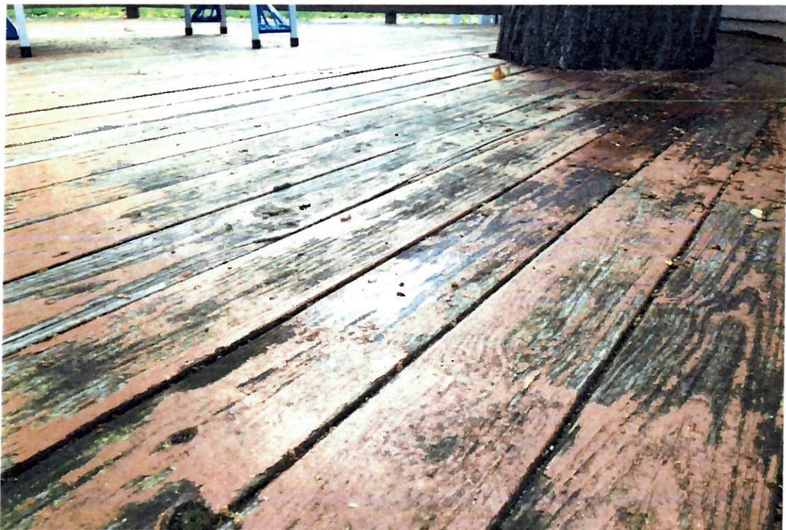
Rotted wood on deck + tree growing into deck
