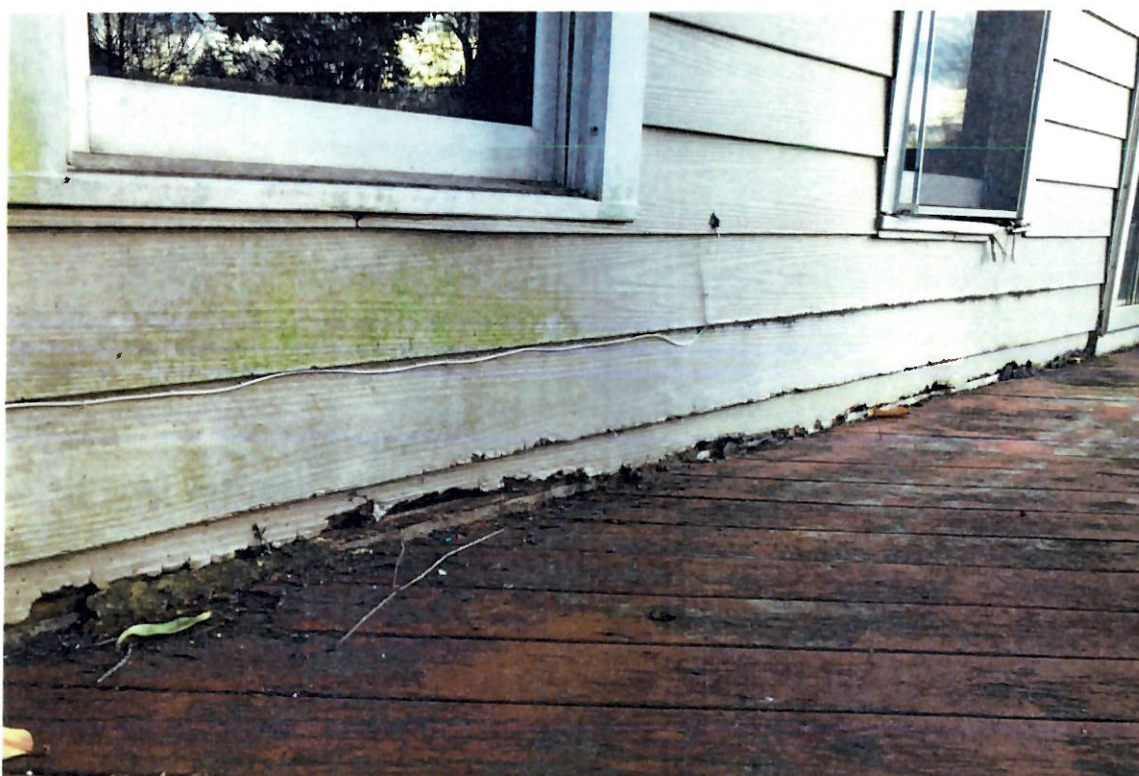
Current deck conditions - rotted wood
