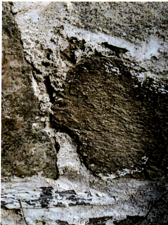
Weathering of mortar around porous stone on front façade.
