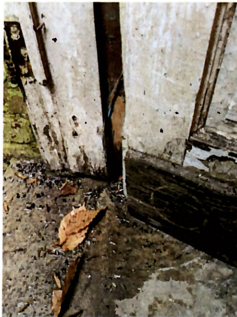
Bottom of right-hand doorframe (as viewed from interior), showing patch installed over rotted door panel and deterioration of wooden doorframe and copper weatherstripping
