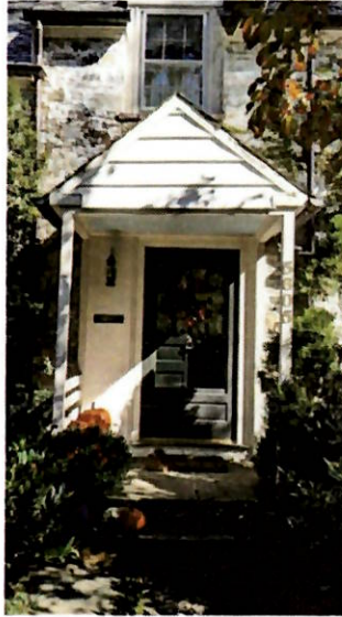
Figure 2. Front porch, showing tilting of roof to left caused by sinking of foundation.
