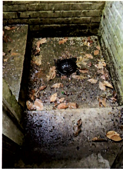
Large catchment basin and dome drain cover installed by current owners to solve basement flooding problem.
