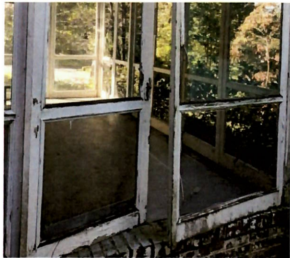
Sagging roof causing screen framing to fail
