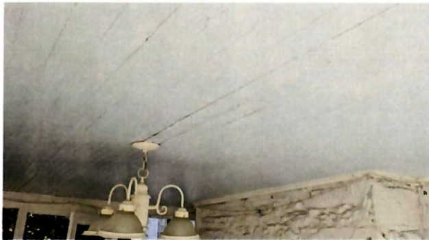
Water damage to ceiling due to failed roof
