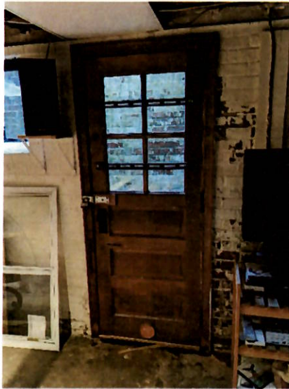
Interior of basement door at bottom of outside steps. Note discoloration at base of doorframe from repeated flooding.
