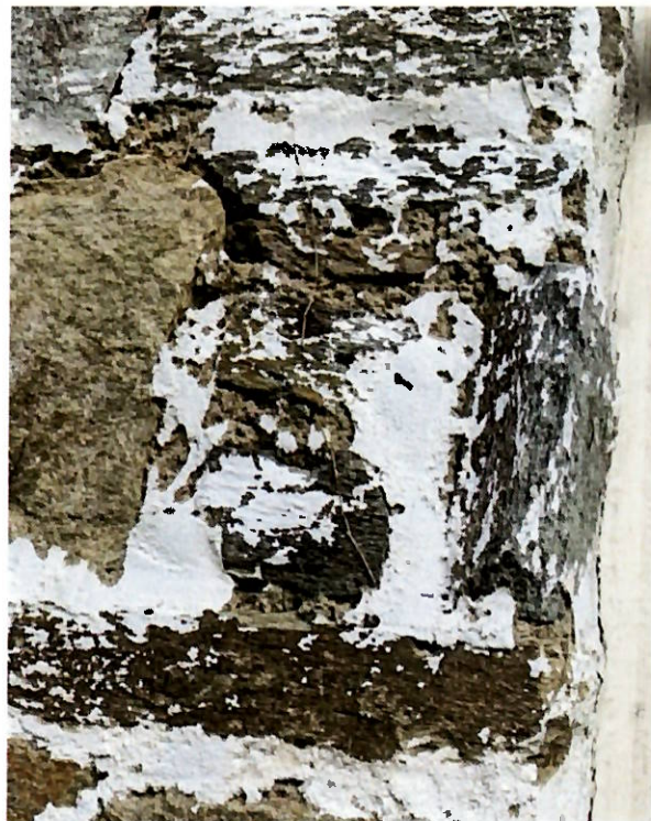
Weathering of mortar around porous stone on front façade.
