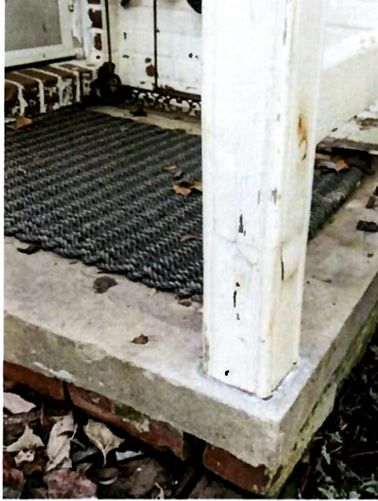
Deteriorating Dutchman installed at base of pillar
