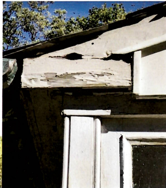
Deterioration of roof members
