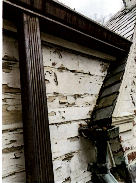
Original ship-lap siding below vinyl siding
