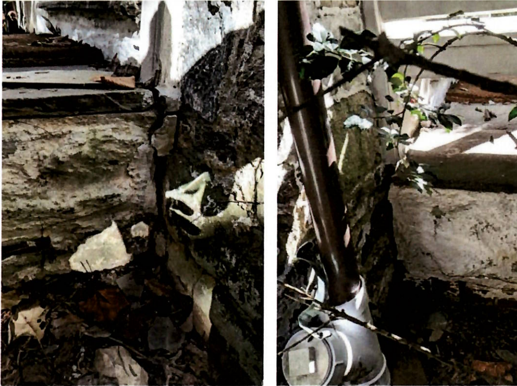
Failure of connection between foundations of house and porch
