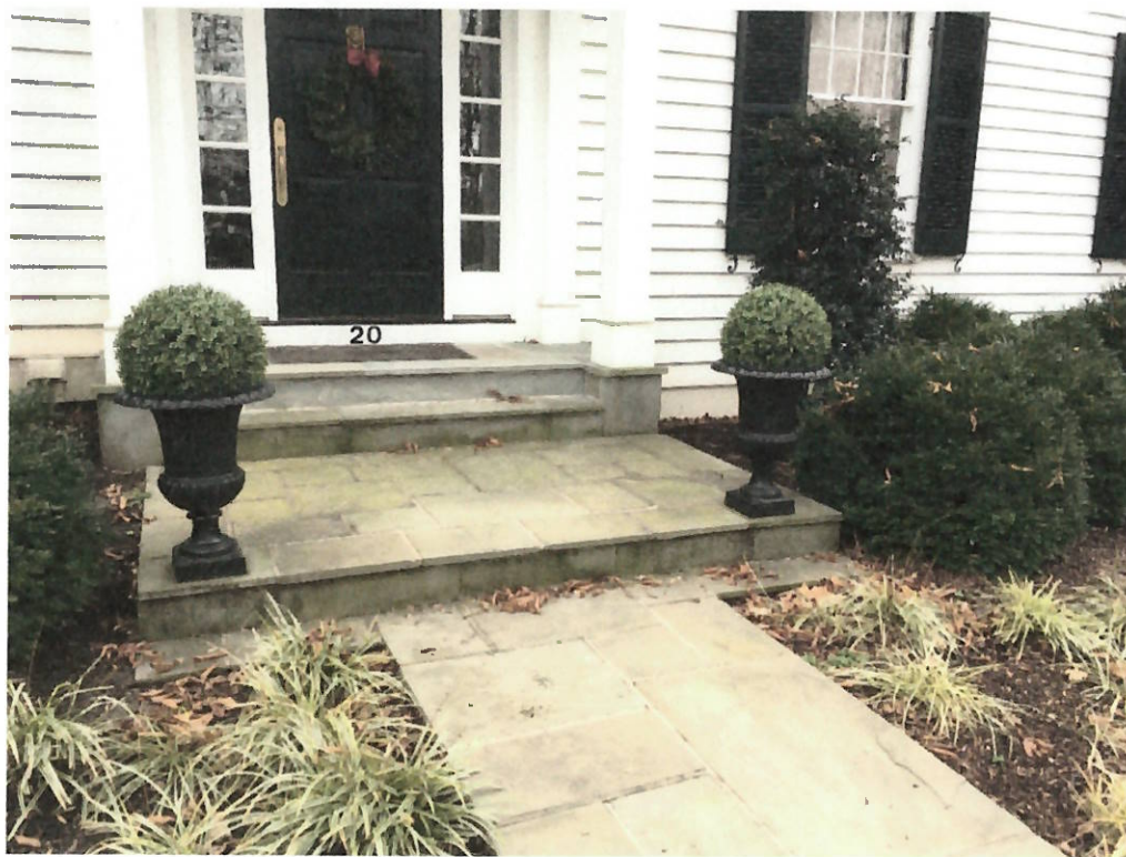
Photo 4- Stoop to be redone to create better landing at door.
