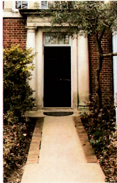
Existing Concrete Walkway Ends at Accessible Entrance. Door does not have an automatic open feature.
