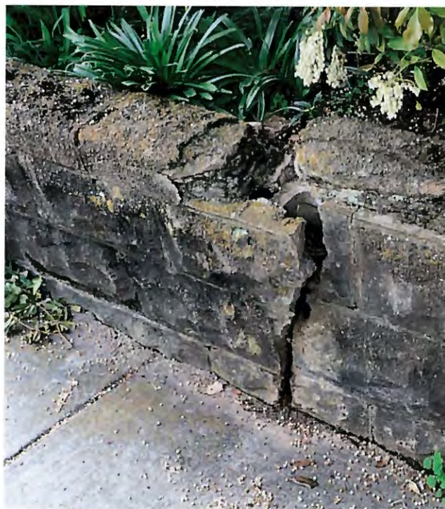
Figure 4—Detail of damage to rusticated cinder block wall
