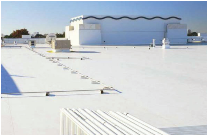
Cool roofs on larger commercial buildings can dramatically reduce energy costs.
