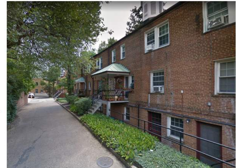
Existing Eastside of Public Alley
