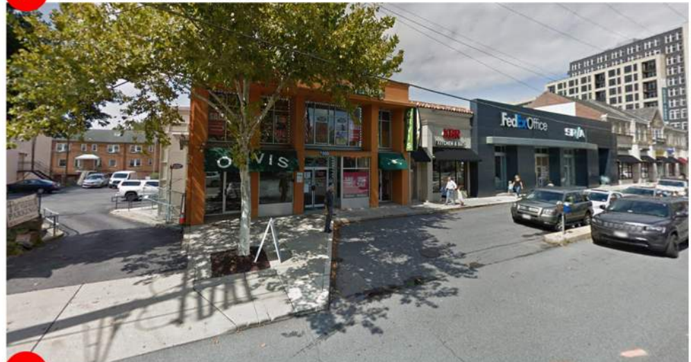
4 NEIGHBORING RETAIL AND LAY-BY STREET PARKING
