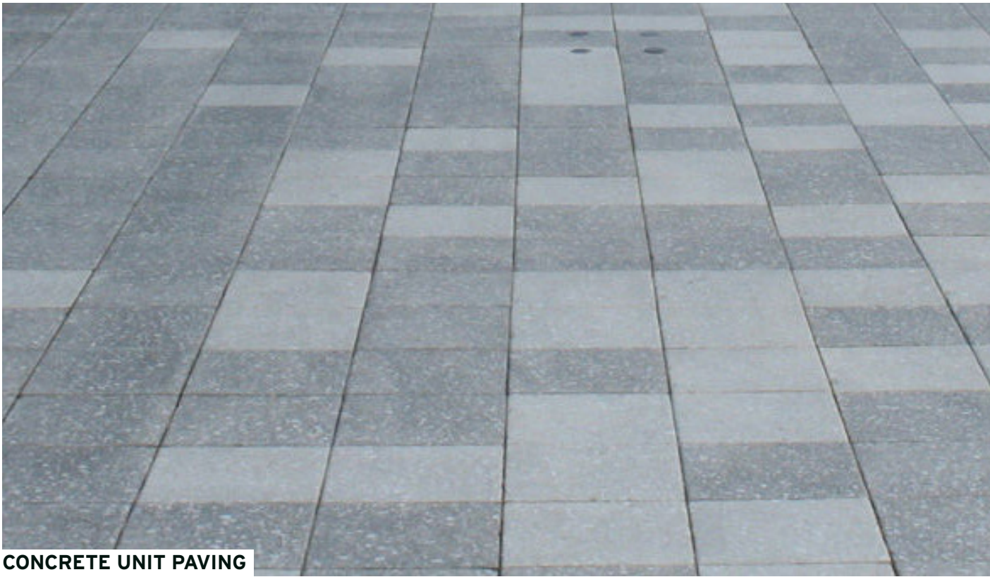
CONCRETE UNIT PAVING
