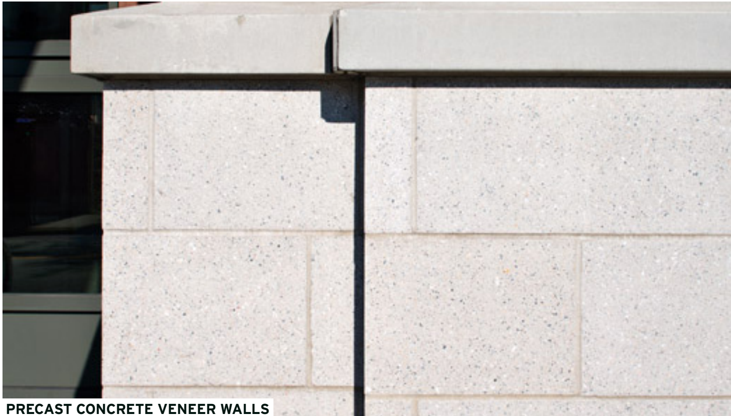
PRECAST CONCRETE VENEER WALLS
