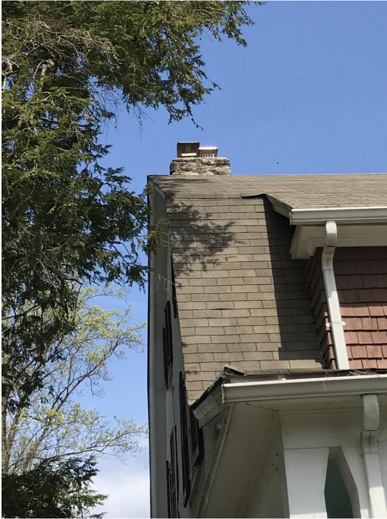
Figure 8: Coal furnace chimney proposed for removal.
