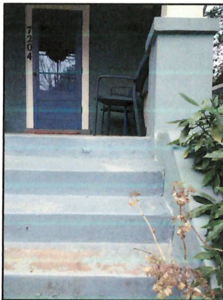
SUBSIDENCE ON RIGHT OF STAIRS
