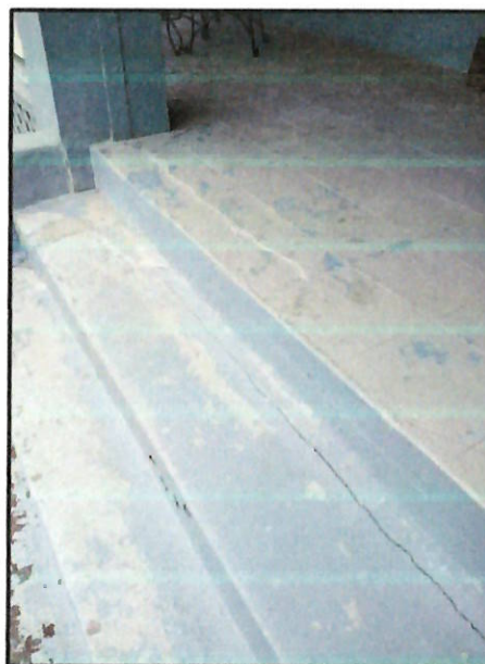
CRACKS ALONG TOP OF STAIRS
