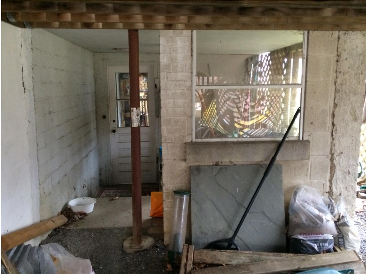
Fig. 3: Photograph from under the existing deck at the northwest corner (rear/left) of the house, looking toward the rear of the house. The concrete block wall of the attached garage is depicted to the left. The location where the alterations will occur is directly above the partially open areaway. Note that the concrete block transitions to parging where the garage was extended.
