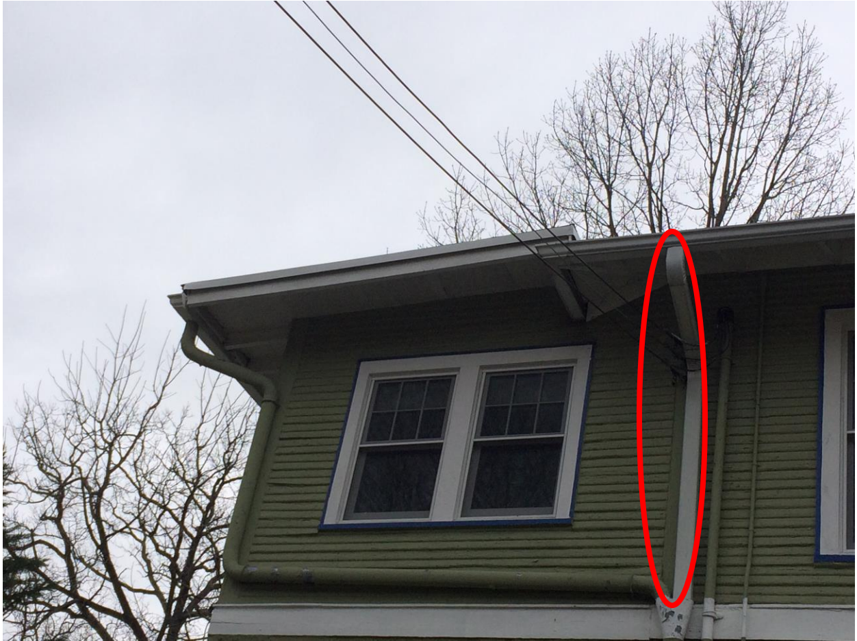
Fig. 7: An original corner board at shown at the transition from the historic house (right) to second-floor of addition (left).
