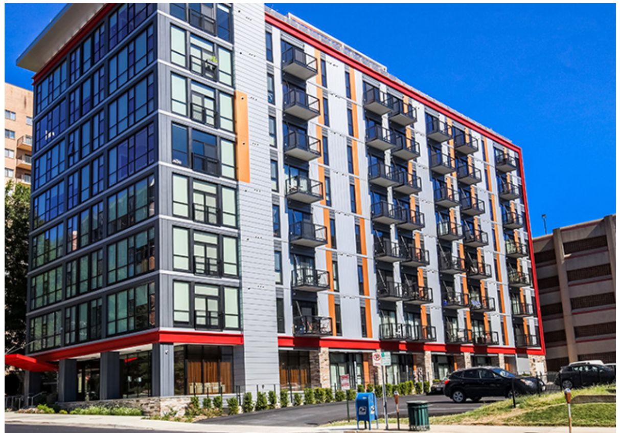
The building facade was reskinned and its scale broken down using balconies, bays, canopies and different architectural materials
