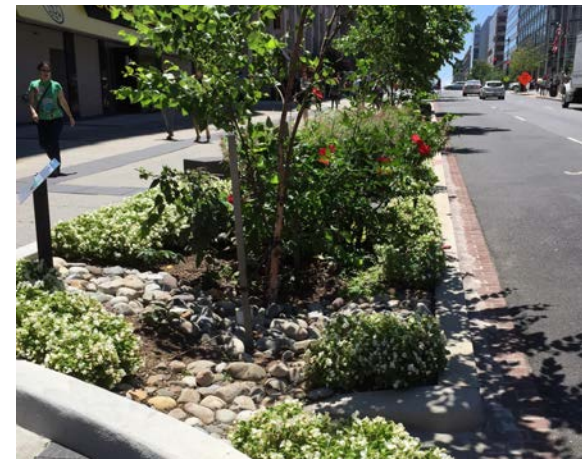
Stormwater management within street design reduces run-off
