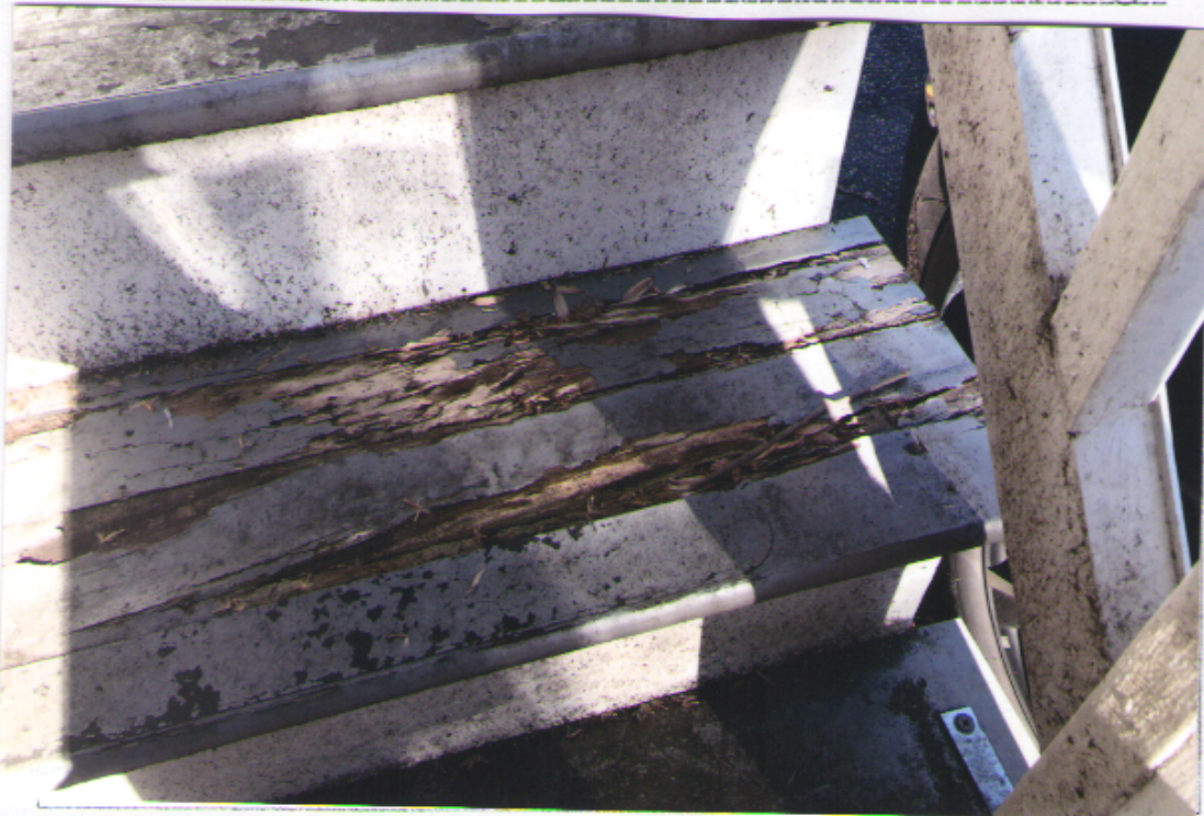
Detail: SIDE PORCH BROKEN/ROTTING STEPS
