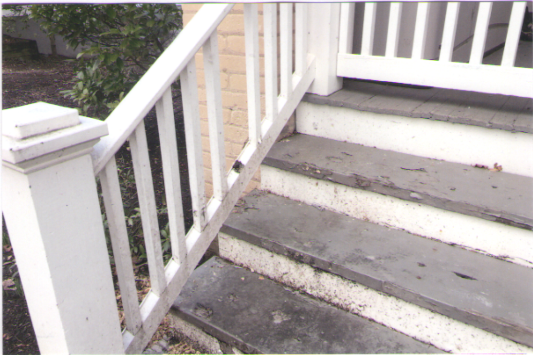
Detail: FRONT PORCH BROKEN RAILING
