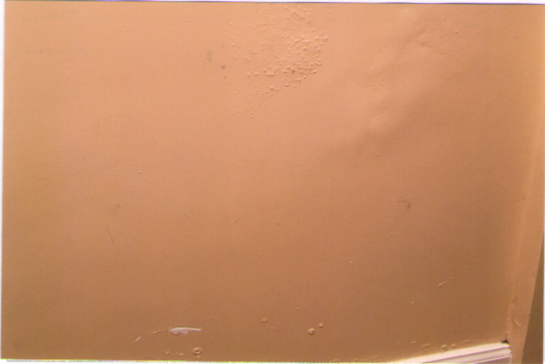
Detail: INTERIOR BASEMENT WATER DAMAGE FROM DOWNSPOUTS
