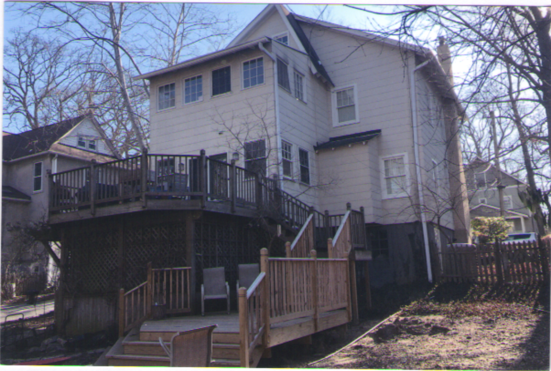
Detail: REAR 1ST+2ND FLOOR ADDITIONS, 1ST FLOOR CLOSET, BACK DECK TO BE REMOVED (SOUTH SIDE VIEW)
