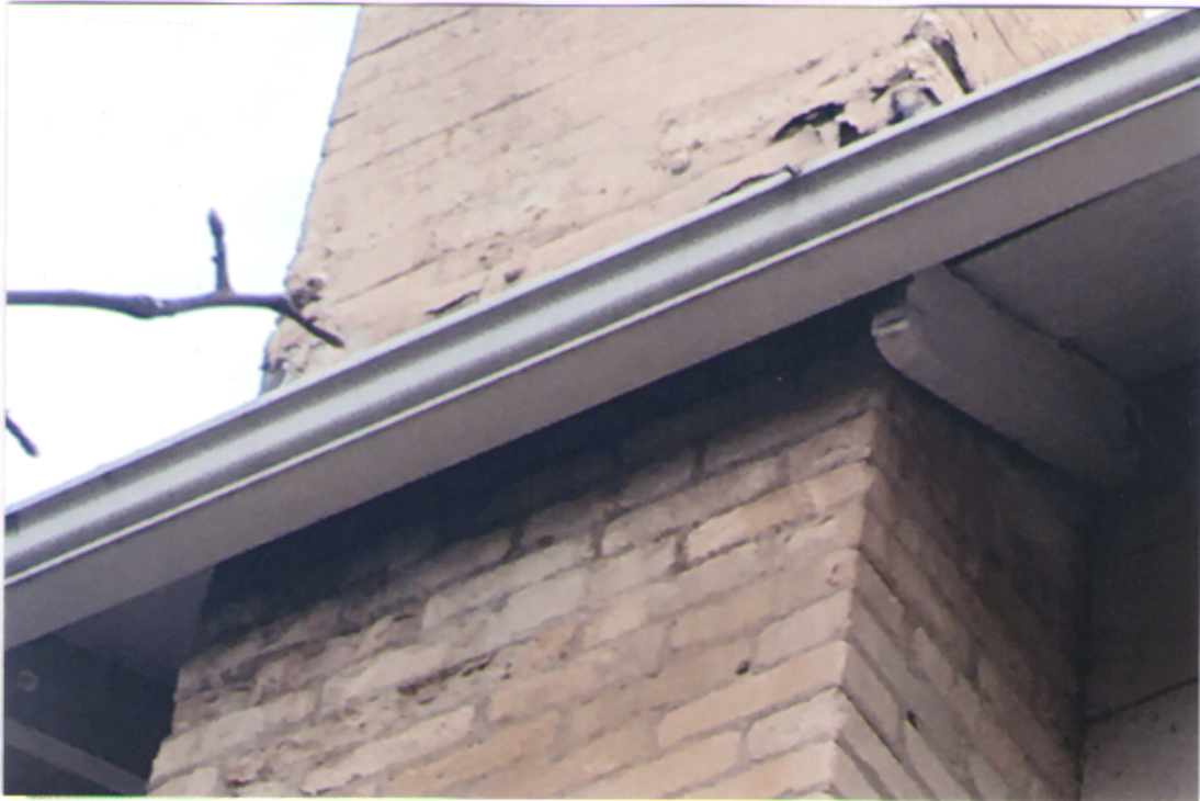
Detail: CHIMNEY DETERIORATING, BROKEN EAVE
