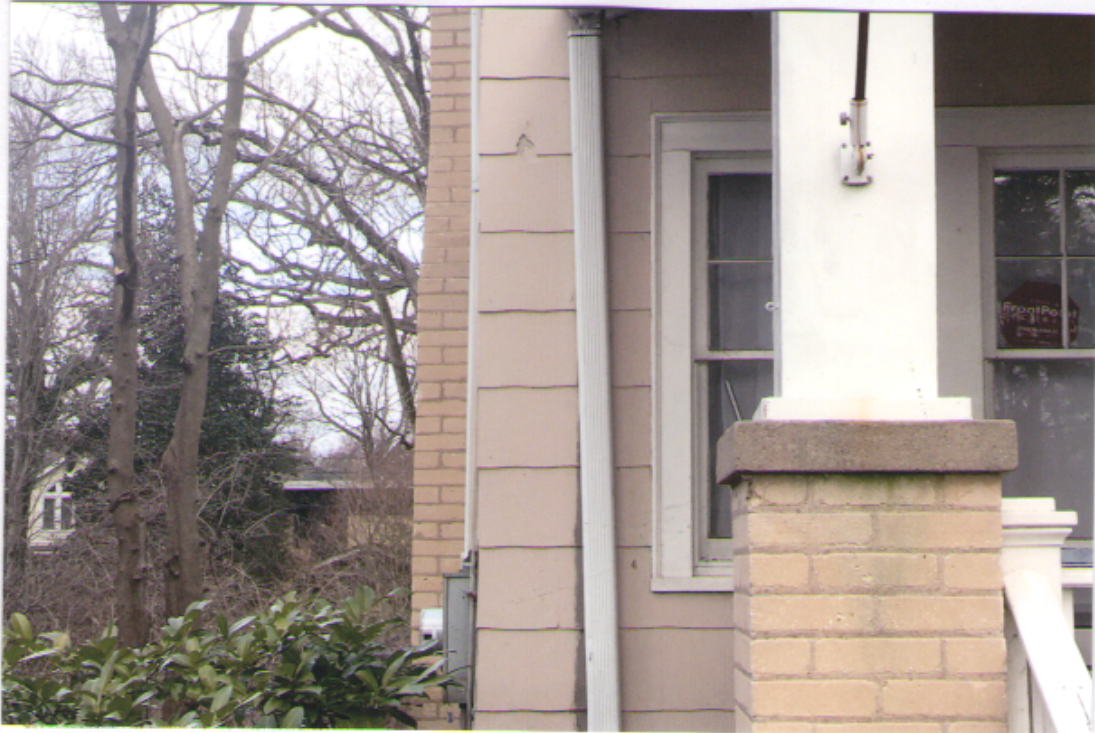
Detail: BROKEN DOWNSPOUTS
