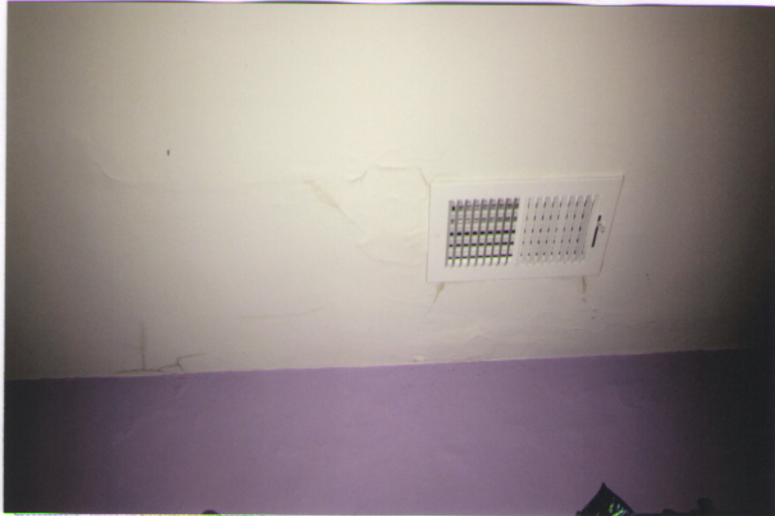
Detail: INTERIOR WATER DAMAGE FROM ROOF, NEAR CHIMNEY
