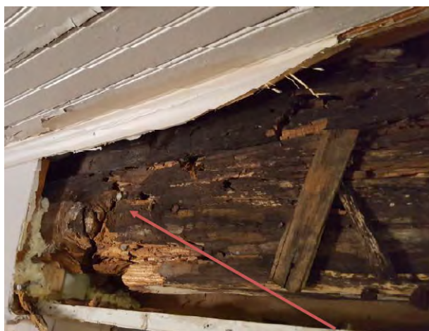
FIGURE 66 Severely deteriorated support beam. Structura, Inc., 2018.
