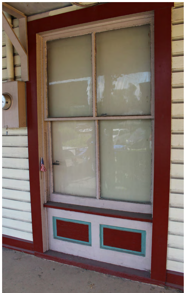
FIGURE 16 Two-over-two wood-sash double hung windows above a solid wood panel with two raised panels.
