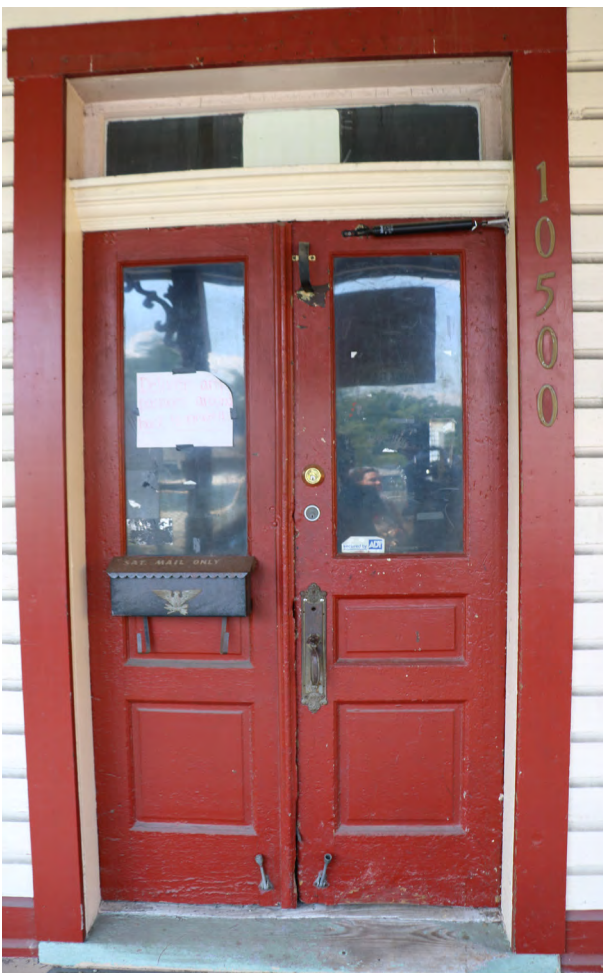
FIGURE 15 Double-leaf doors with two raised wood panels.
