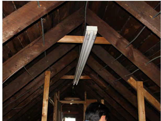
FIGURE 62 Gable roof framing.
