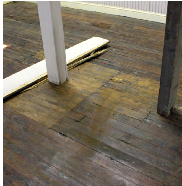
FIGURE 84 Interior, wood plank flooring transition from original construction to south wing.
