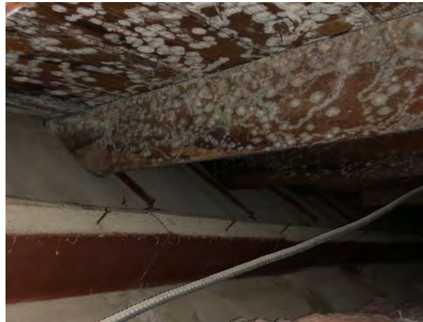
FIGURE 69 Termite damage and mold on the underside of north wing roof framing. Structura, Inc., 2019.
