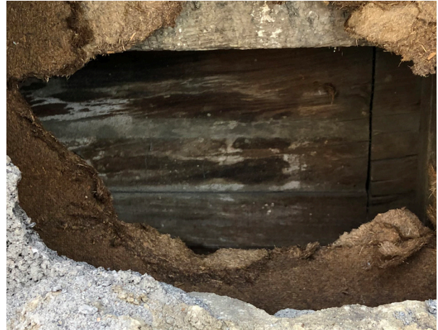
FIGURE 23 Exploratory demolition revealed wood siding in poor condition on west elevation. Antunovich Associates, 2019.
