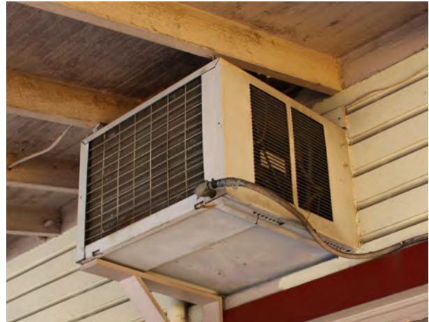
FIGURE 36 Through wall AC unit at front facade.
