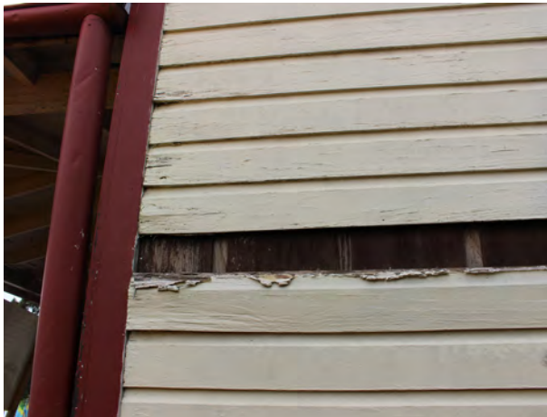
FIGURE 31 Missing German lap siding that reveals the extant vertical siding.
