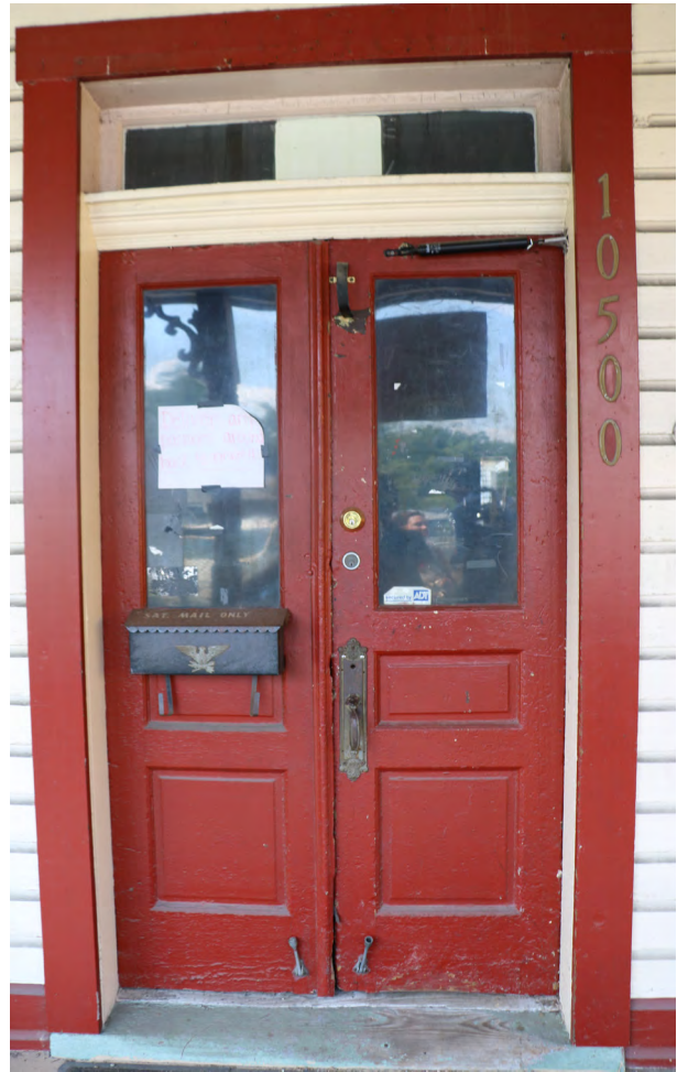
FIGURE 55 Double-leaf doors with two raised wood panels.
