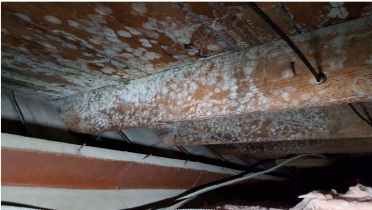
18. Low roof joists on north wing of building with significant mold growth.
