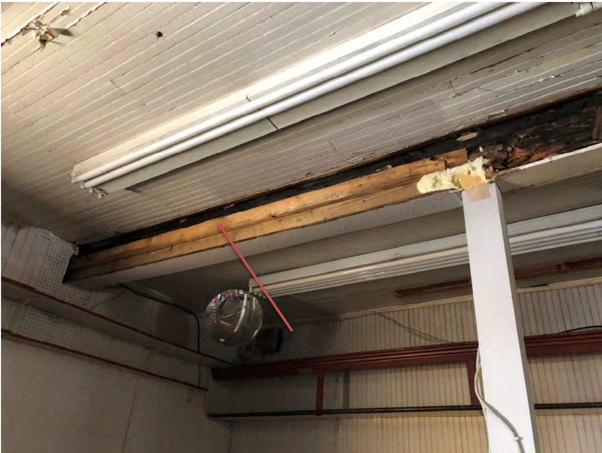
16. New wood beam placed at south wing of building.
