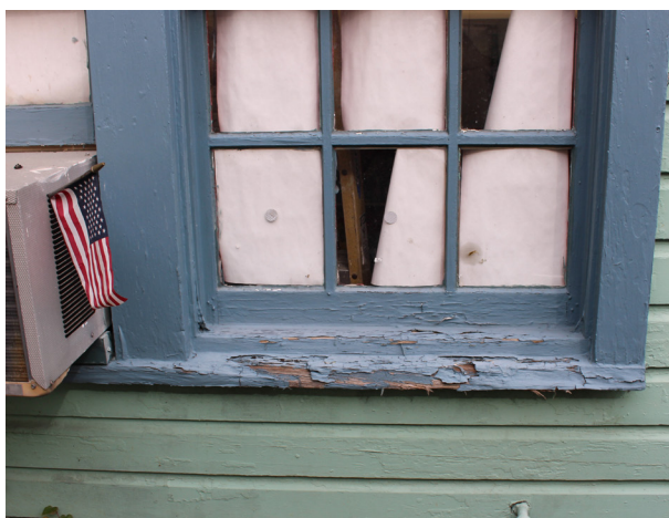
FIGURE 22 Deteriorated sill, south elevation.
