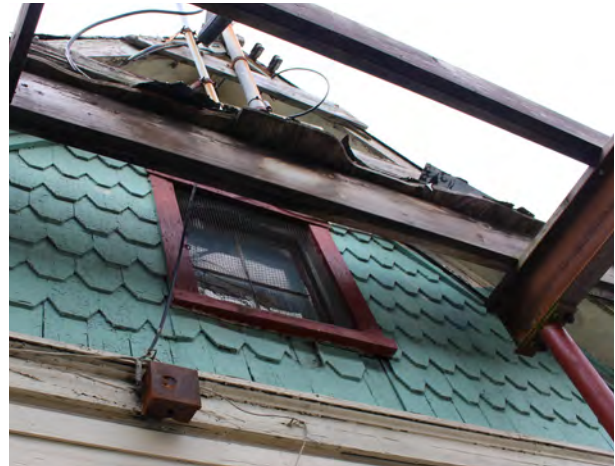
FIGURE 35 Trapezoidal-cut shingles on north gable.
