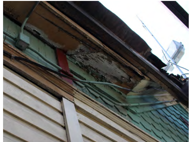
FIGURE 44 Deteriorated eve condition.
