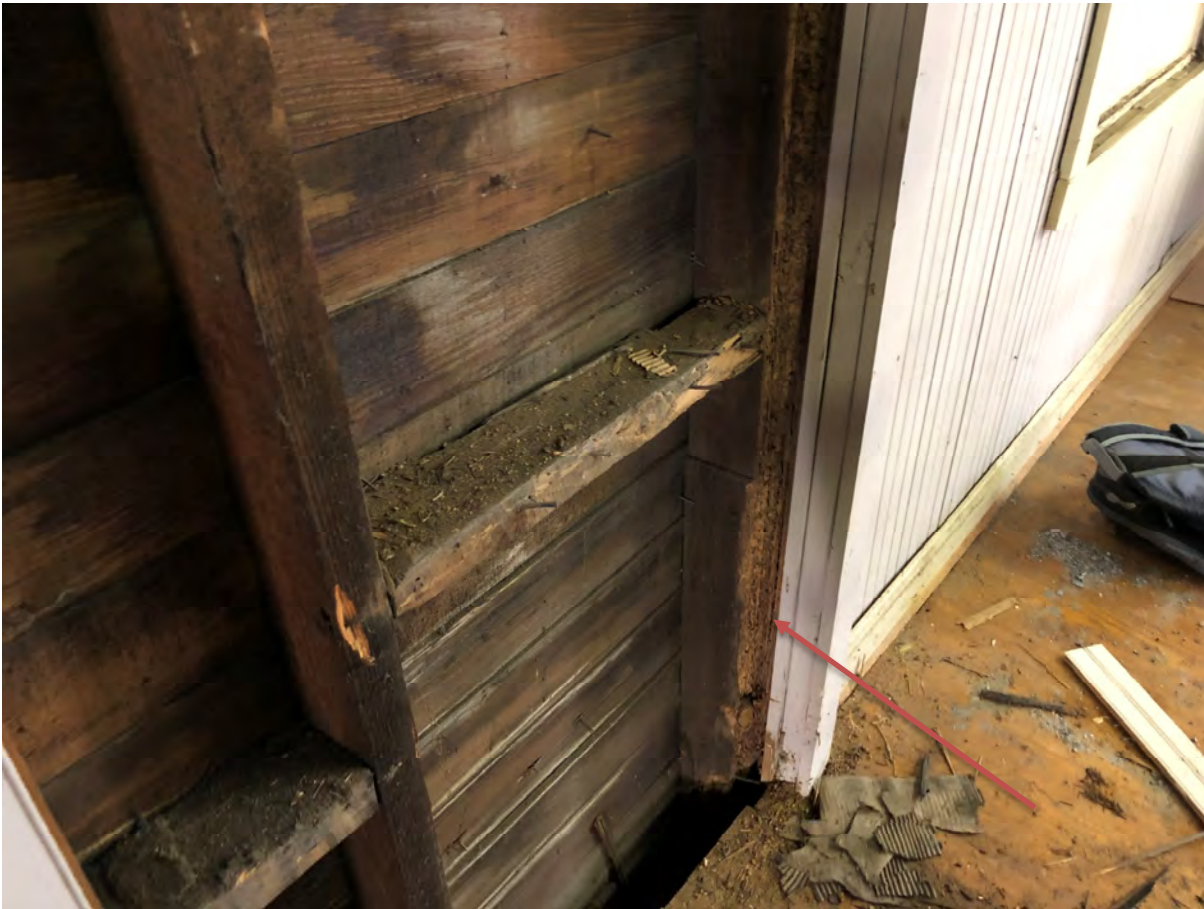
17. Termite damage to wood post on south wall of building.
