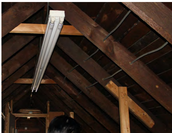
FIGURE 70 Sistered roof framing.
