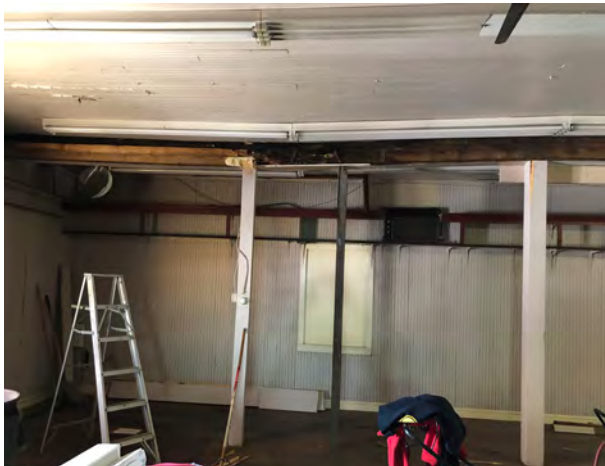
FIGURE 61 Deteriorated wood beam and interior columns. Structura, Inc., 2019.
