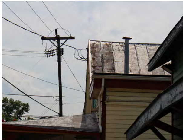
FIGURE 43 Rust and deterioration of metal sheathing visible on center gable.
