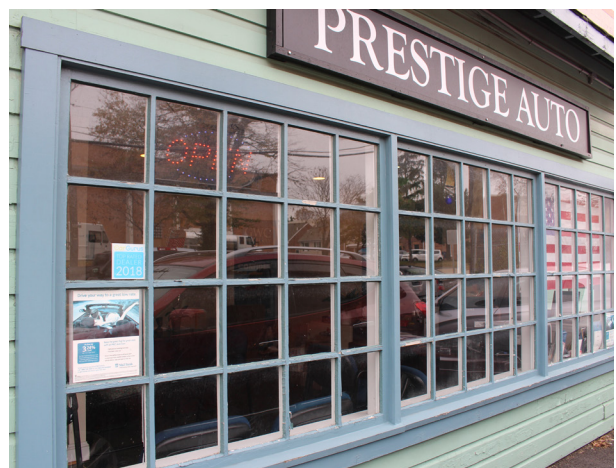
FIGURE 25 Non-original multi-light windows, north elevation, in generally good condition.
