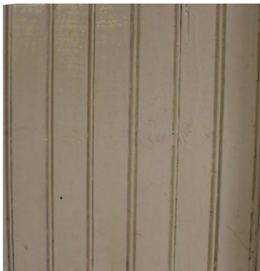
FIGURE 88 Interior, typical beadboard at walls and ceiling.
