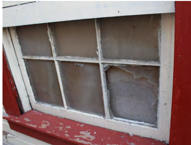
FIGURE 47 Broken glazing.
