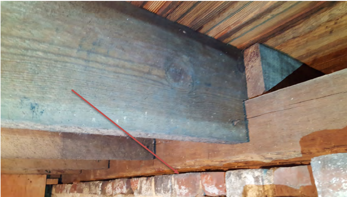
13. Existing joists notched at support. Sill plate is not fully bearing on foundation wall.
