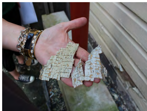
FIGURE 33 Flaking paint.
