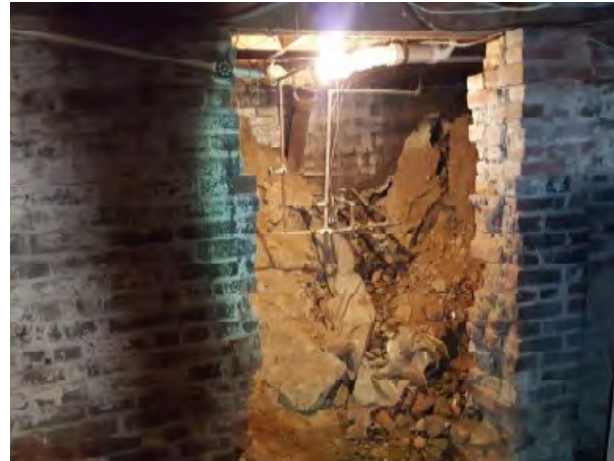
FIGURE 64 Opening demolished in section of foundation wall. Structura, Inc., 2018.
