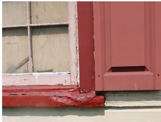
FIGURE 48 Sill deterioration.
