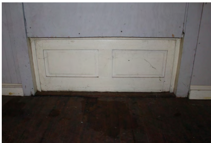
FIGURE 75 Simple trim and wood panels below facade windows.
