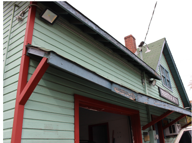
FIGURE 24 Deteriorated, non-original, shed canopy.
