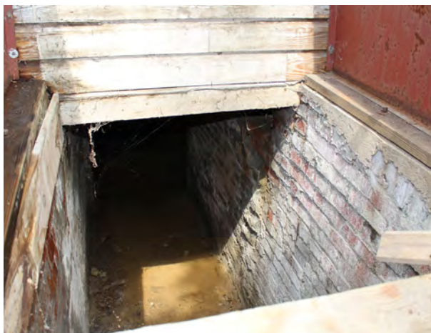
FIGURE 37 Brick foundation walls visible at basement access hatch.
