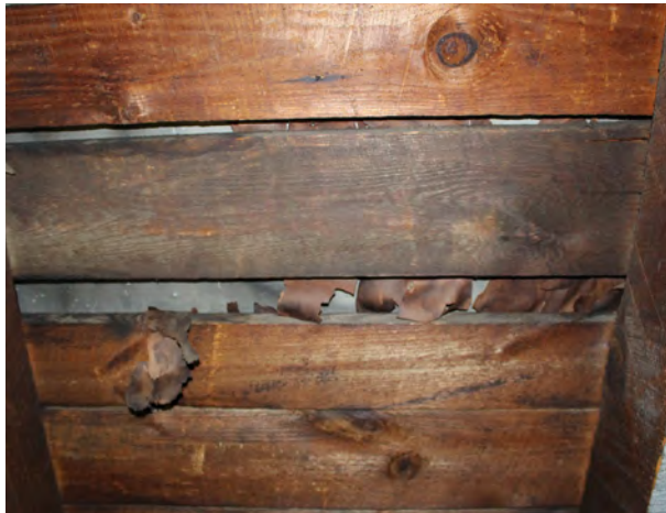
FIGURE 68 Deteriorated roof sheathing.
