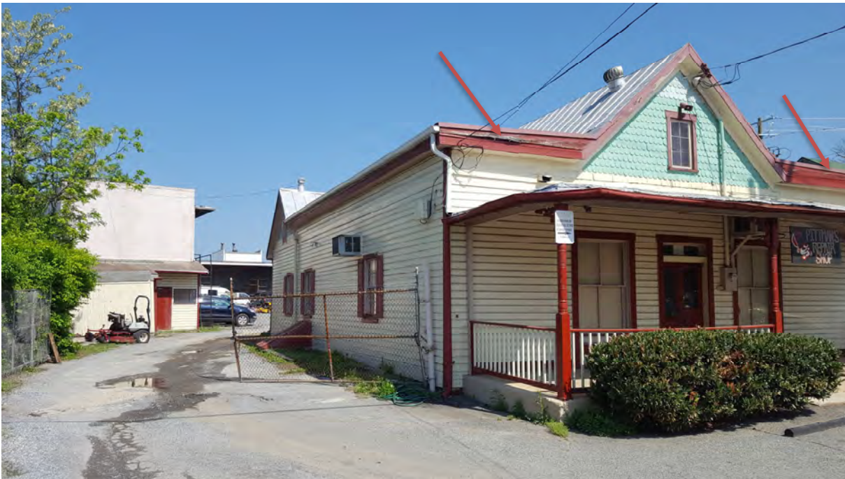
22. Low roof framing appears to have been over-built over existing roof framing on north and south wings of building.
