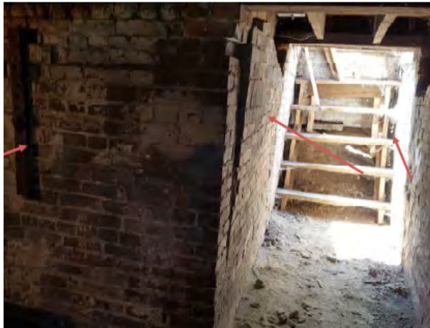
FIGURE 63 Laterally displaced foundation wall, undermined footing below access hatch and stair, and previous foundation wall retrofit. Structura, Inc., 2018.
