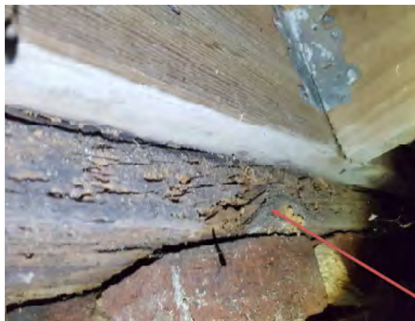
FIGURE 67 Replacement wood joist framing. Wood ledge connected to original wood sill plate that exhibits insect damage. Joist and ledger are not adequately connected. Structura, Inc., 2018.
