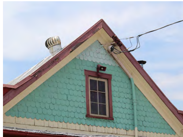
FIGURE 29 Decorative shingles on end gable, east elevation.
