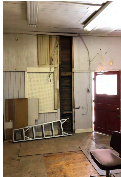
FIGURE 87 Interior, various layers of wall cladding materials revealed during exploratory demolition.
