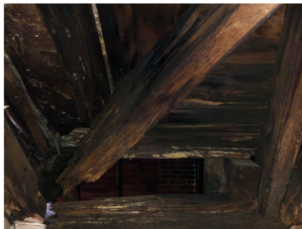
FIGURE 71 Deteriorated roof framing. Structura, Inc., 2019.
