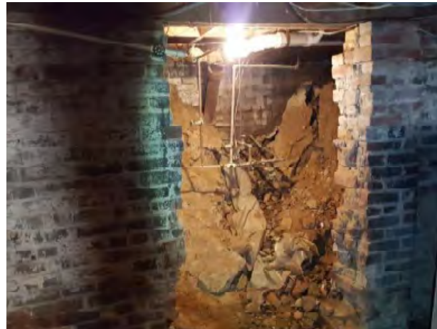
FIGURE 58 Opening in section of foundation wall. Structura, Inc., 2018.
