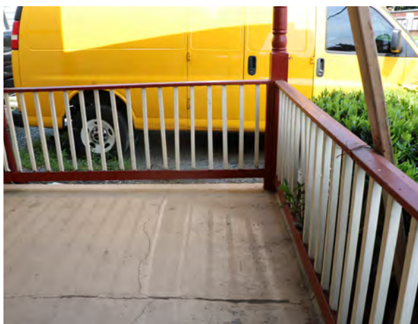
FIGURE 41 Cracks in concrete slab.
