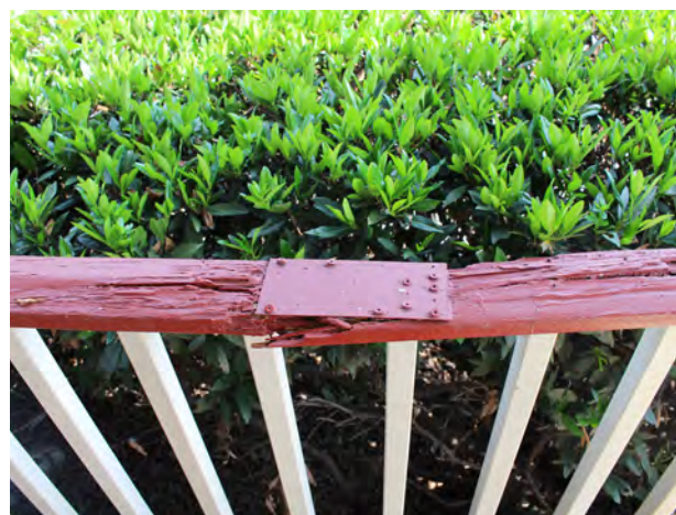
FIGURE 42 Splintered banister (non-original).
