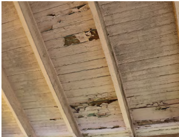
FIGURE 39 Deteriorated porch ceiling.
