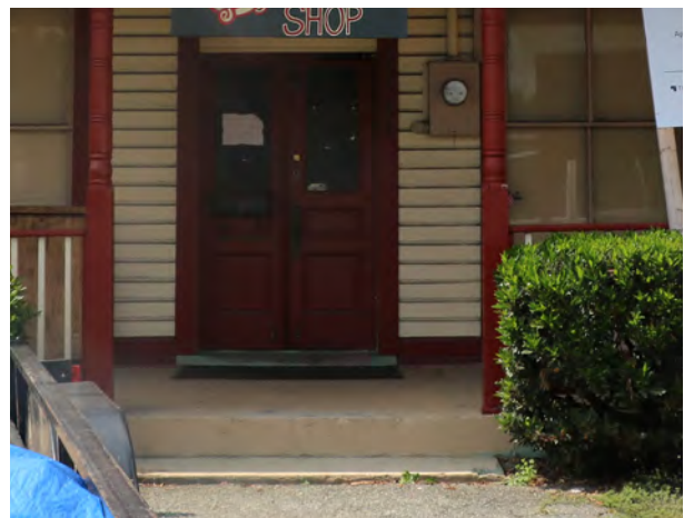
FIGURE 38 Painted concrete porch and step.
