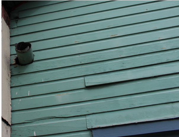
FIGURE 20 Detail, wood siding, loose boards.
