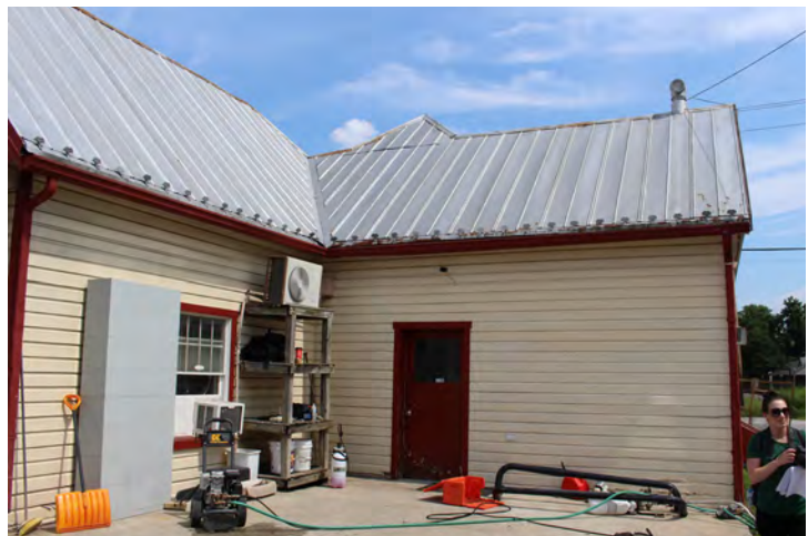
FIGURE 23 Concrete slab, non-original door on 1927 rear addition.
