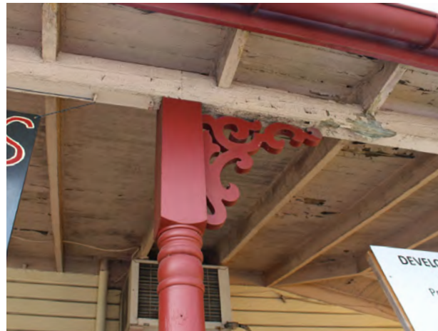
FIGURE 40 Non-original porch posts and decorative brackets.
