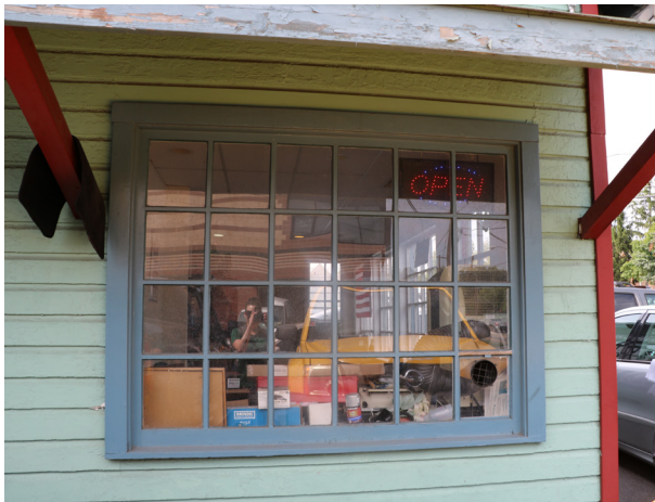
FIGURE 16 Non-original multi-light window, east elevation.
