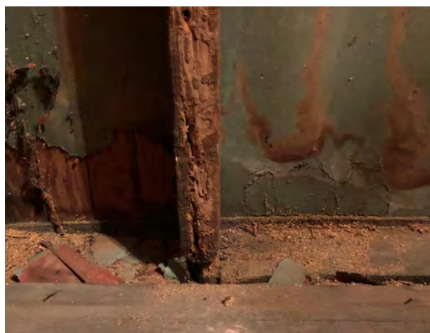
FIGURE 65 Termite damage visible in wall framing. Structura, Inc., 2019.
