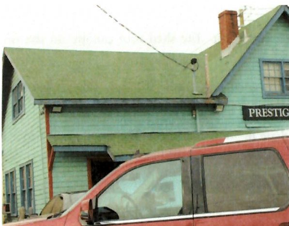
FIGURE 21 Asphalt shingle roof appears to be in generally good condition.
