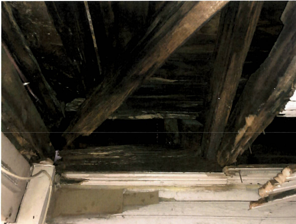
19. Deteriorated low roof framing on south wing of building.
