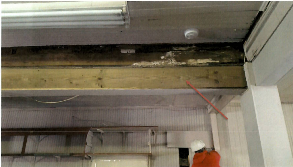
15. New wood beam placed below deteriorated wood beam on south wing of building.
