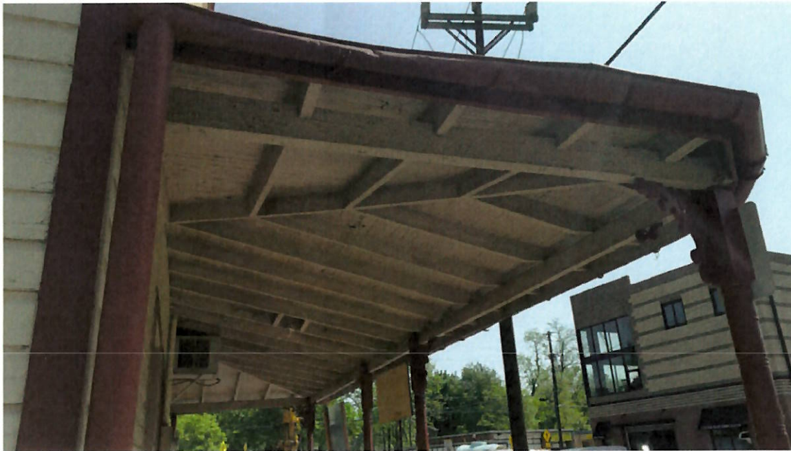
21. Existing porch roof framing
