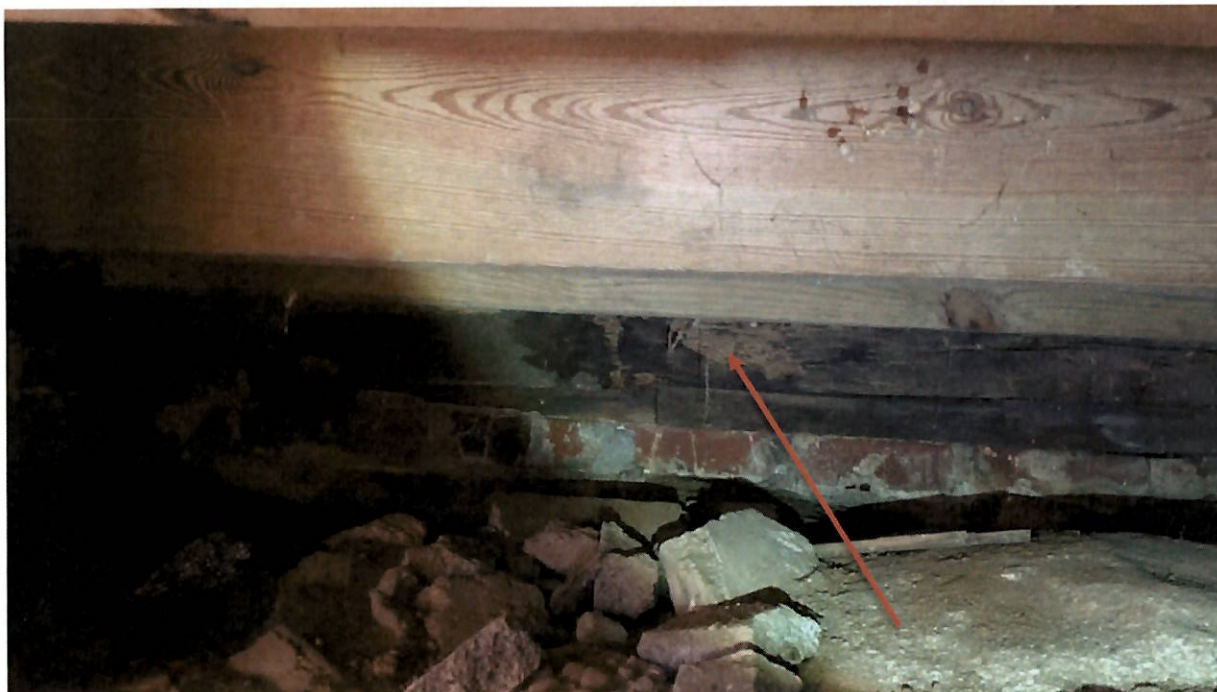
12. Replacement wood joists. Note existing joist remaining that appears to have damage from wood destroying insects.
