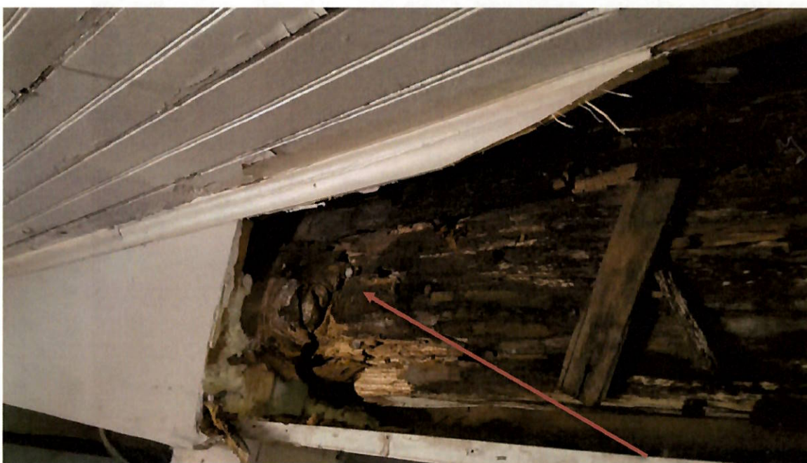
14. Severely deteriorated wood beam supporting roof framing on south wing of building.
