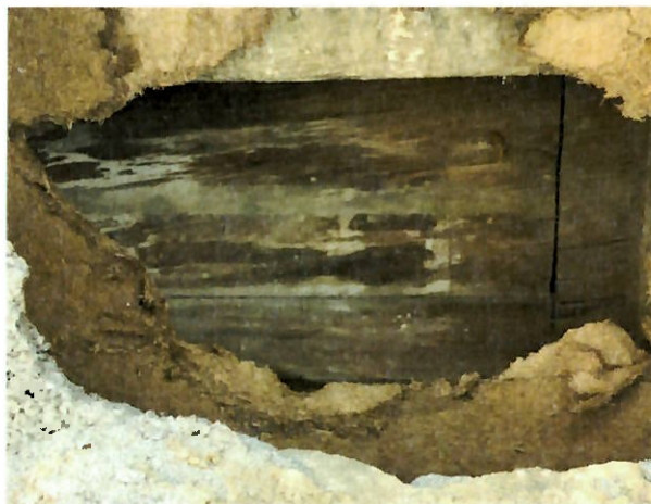
FIGURE 23 Exploratory demolition revealed wood siding in poor condition on west elevation. Antunovich Associates, 2019.
