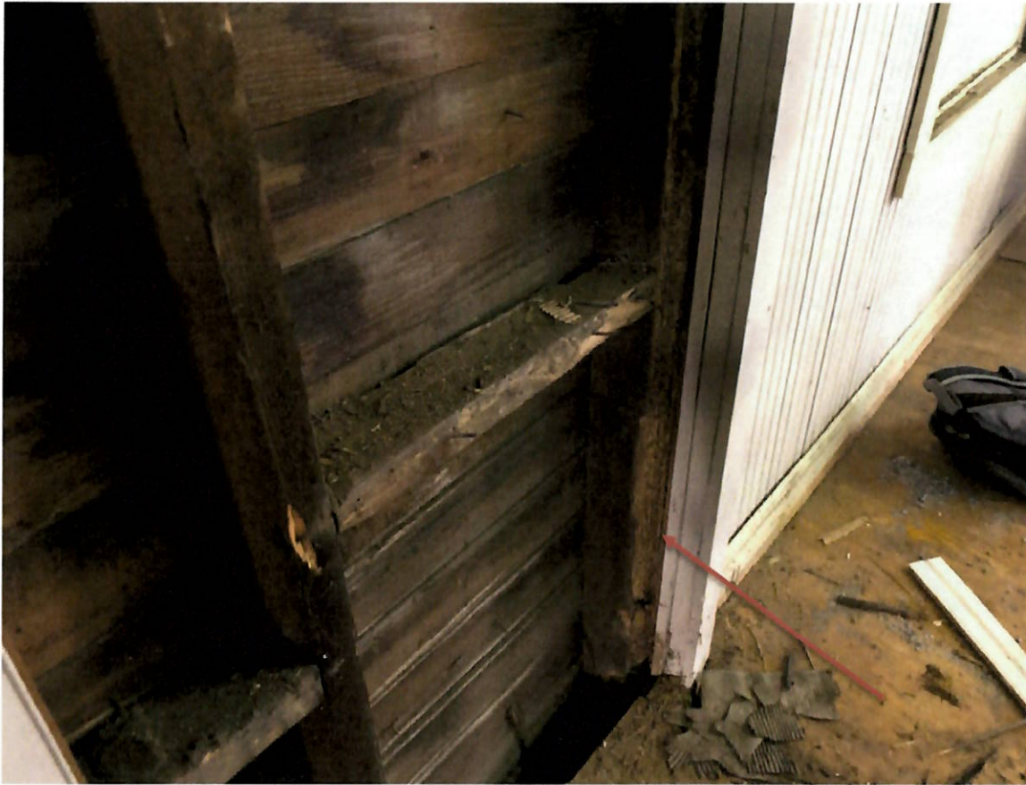
17. Termite damage to wood post on south wall of building.
