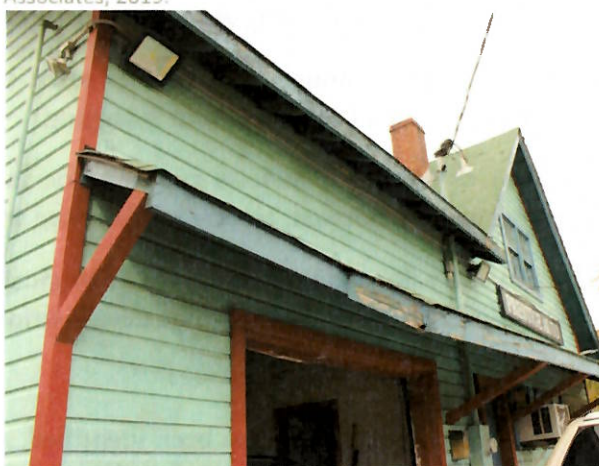
FIGURE 24 Deteriorated, non-original, shed canopy.
