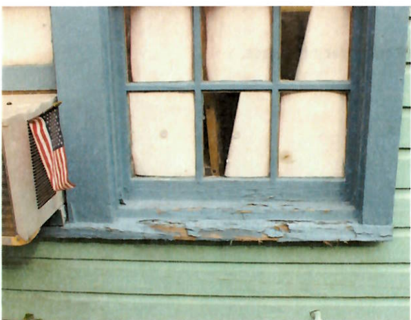
FIGURE 22 Deteriorated sill, south elevation.
