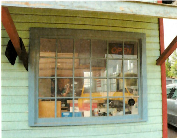
FIGURE 16 Non-original multi-light window, east elevation.
