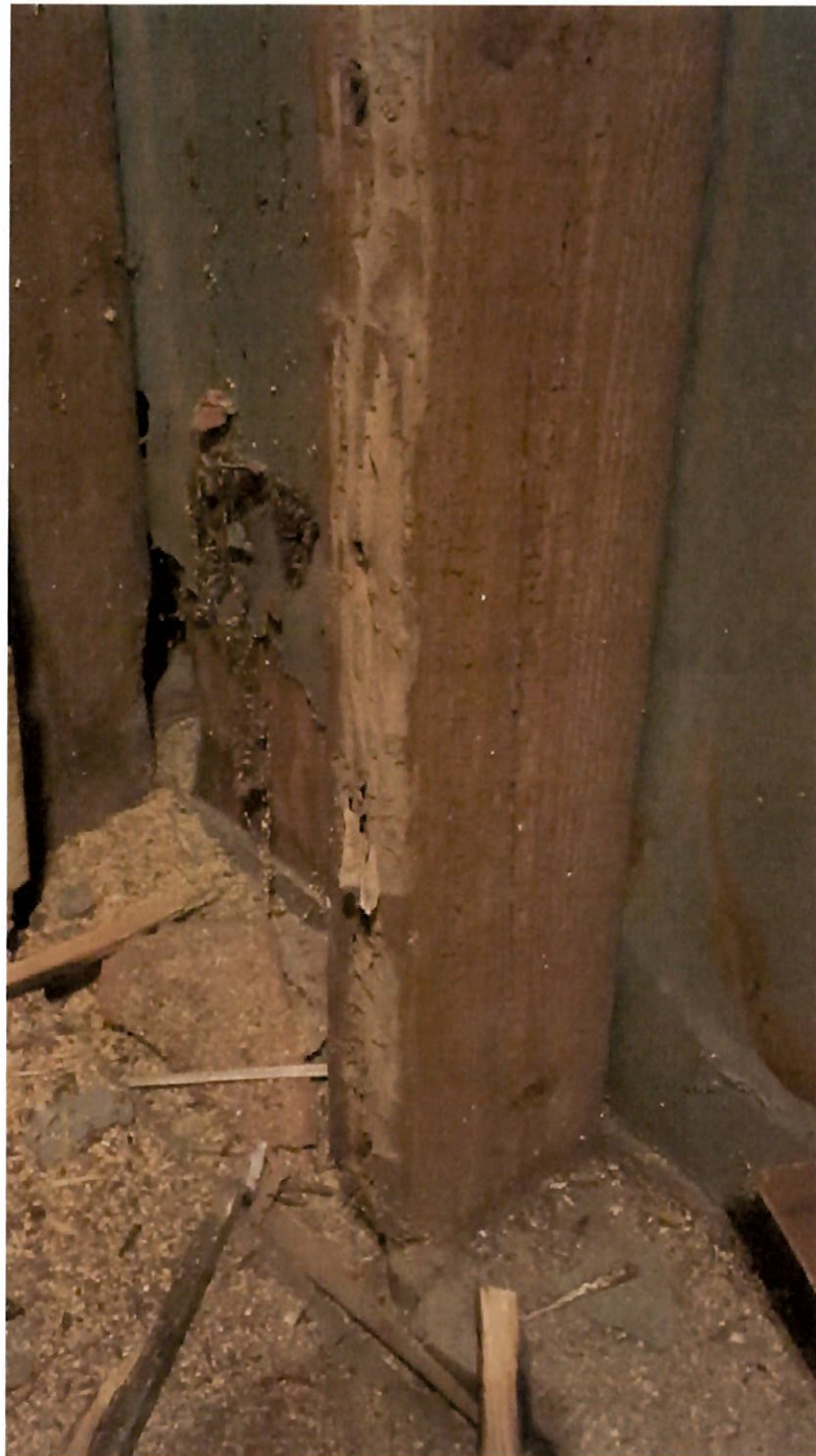
20. Termite damage to existing wall stud at interior load bearing wall on north wing of building.
