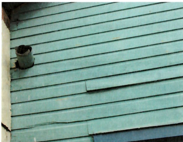
FIGURE 20 Detail, wood siding, loose boards.
