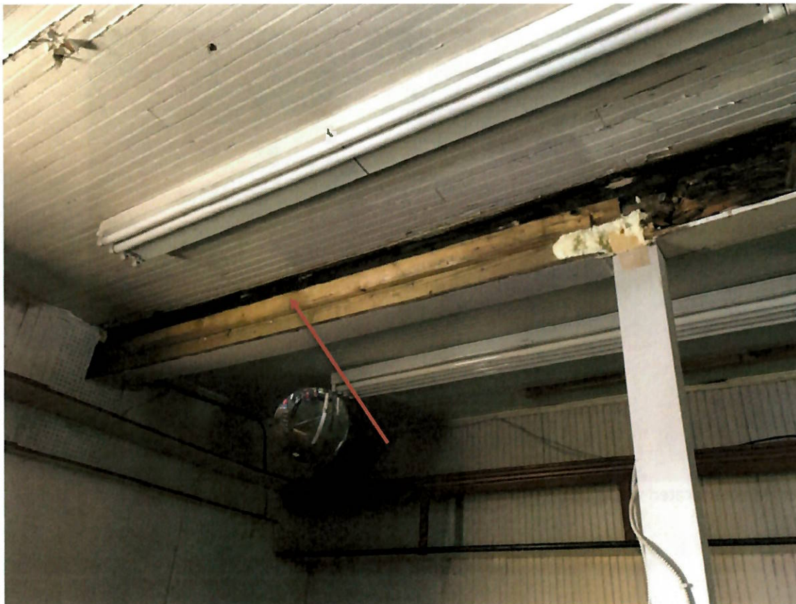
16. New wood beam placed at south wing of building.
