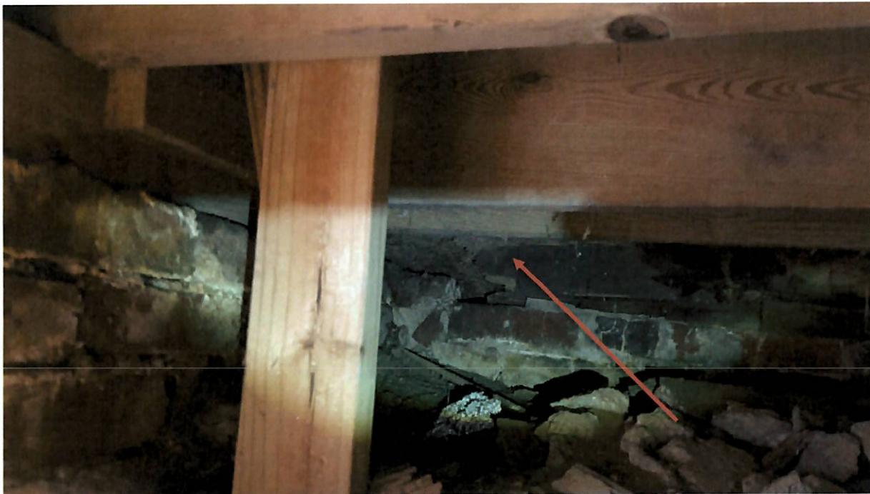
11. Original band joist still in place appears to have been damaged by wood destroying insects.
