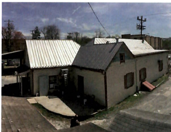
FIGURE 46 Contemporary metal roofing visible on rear addition.
