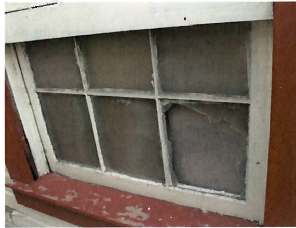
FIGURE 47 Broken glazing.
