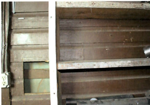
FIGURE 76 Interior, original exterior painted wood siding, extant within north wing storage space.
