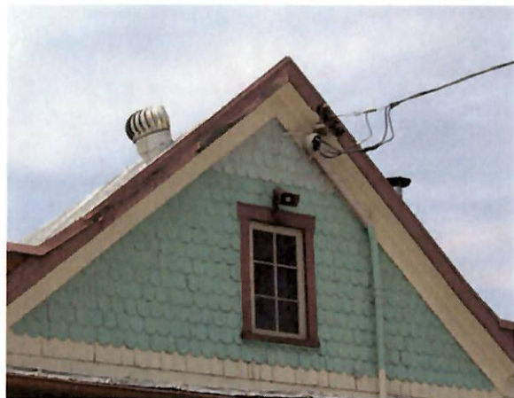
FIGURE 29 Decorative shingles on end gable, east elevation.
