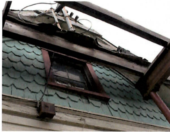
FIGURE 35 Trapezoidal-cut shingles on north gable.
