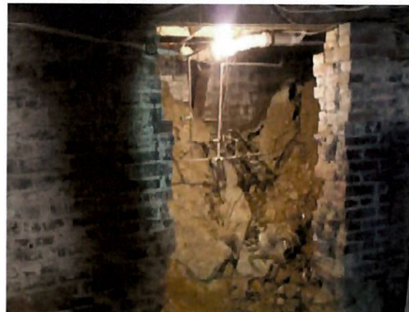
FIGURE 64 Opening demolished in section of foundation wall. Structura, Inc., 2018.
