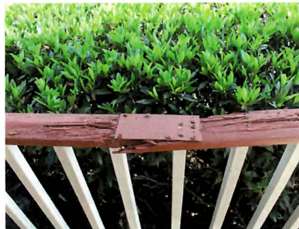
FIGURE 42 Splintered banister (non-original).
