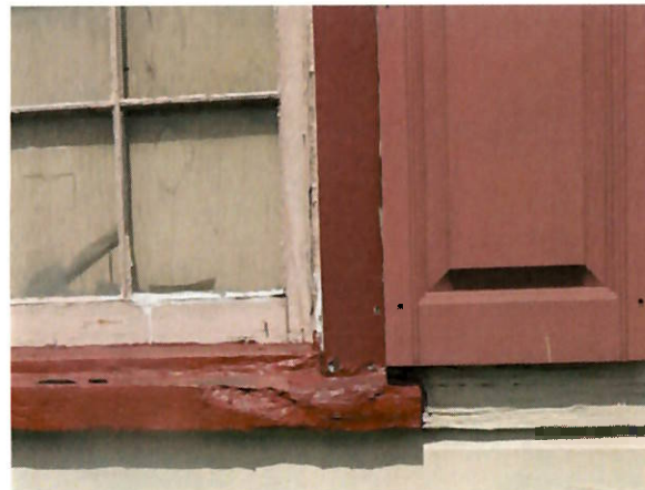
FIGURE 48 Sill deterioration.
