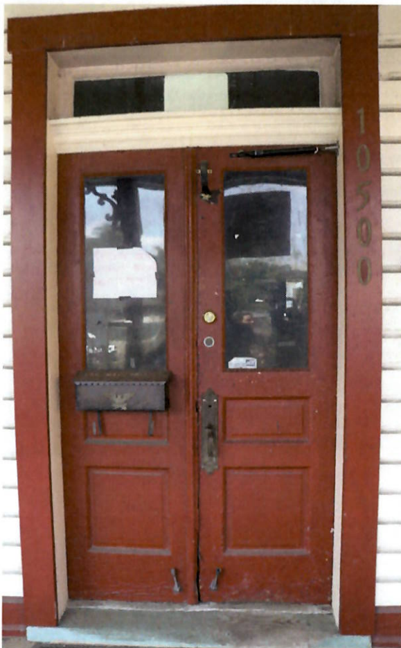
FIGURE 15 Double-leaf doors with two raised wood panels.
