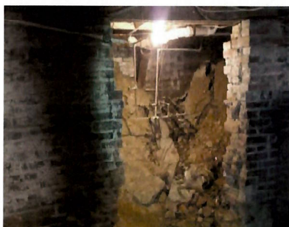
FIGURE 58 Opening in section of foundation wall. Structura, Inc., 2018.
