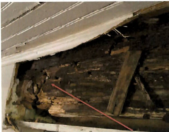
FIGURE 66 Severely deteriorated support beam. Structura, Inc., 2018.
