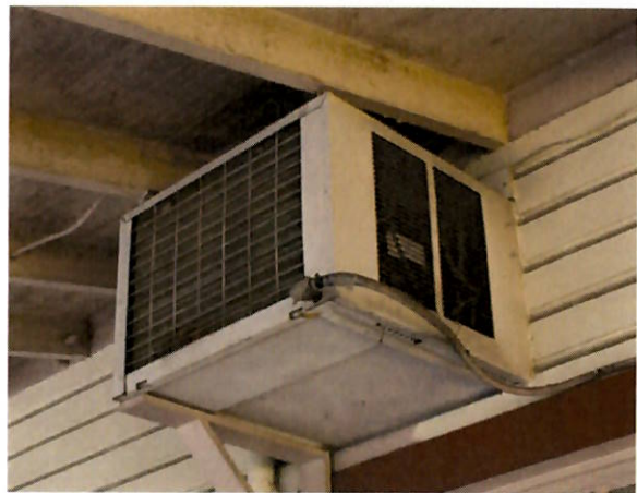
FIGURE 36 Through wall AC unit at front facade.
