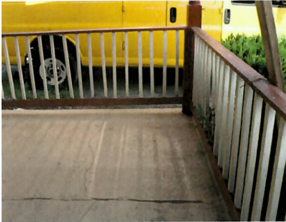
FIGURE 17 Crack in concrete slab; non-original wood balusters and banister.
