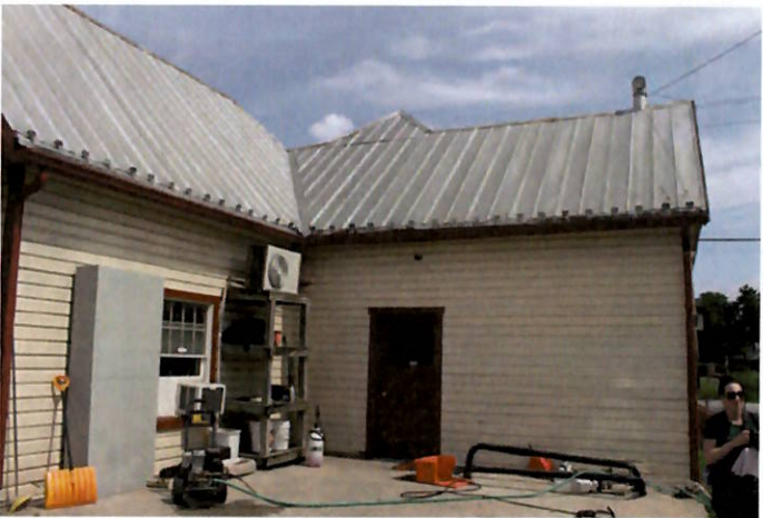
FIGURE 23 Concrete slab, non-original door on 1927 rear addition.
