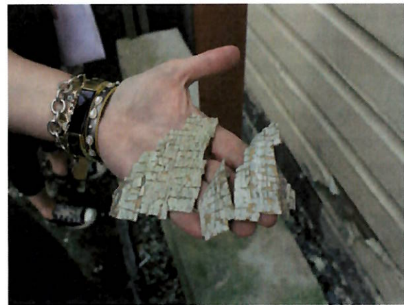
FIGURE 33 Flaking paint.
