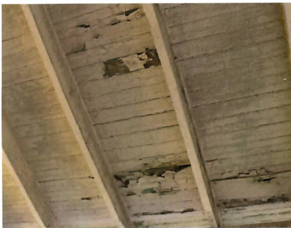
FIGURE 39 Deteriorated porch ceiling.
