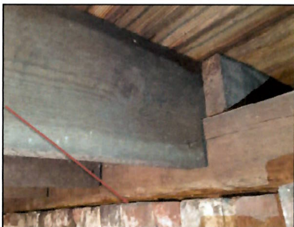
FIGURE 59 Sill plate not fully bearing on foundation wall. Structura, Inc., 2018.
