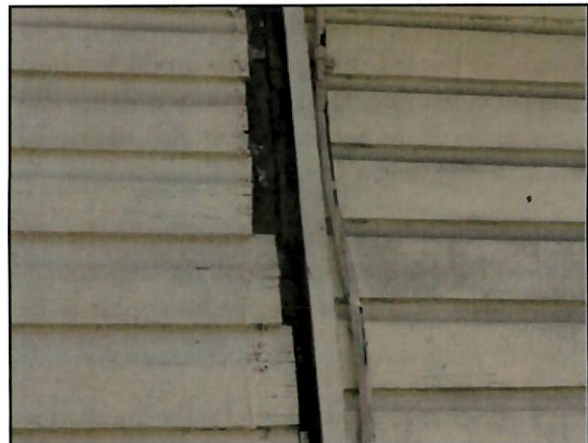
FIGURE 34 Missing portion of wood siding, exposed framing, north elevation.
