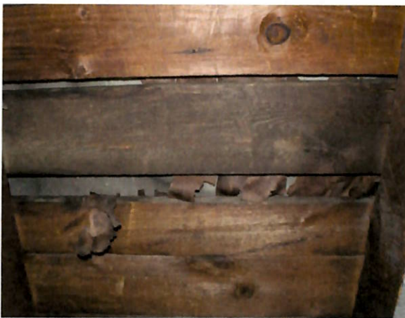
FIGURE 68 Deteriorated roof sheathing.
