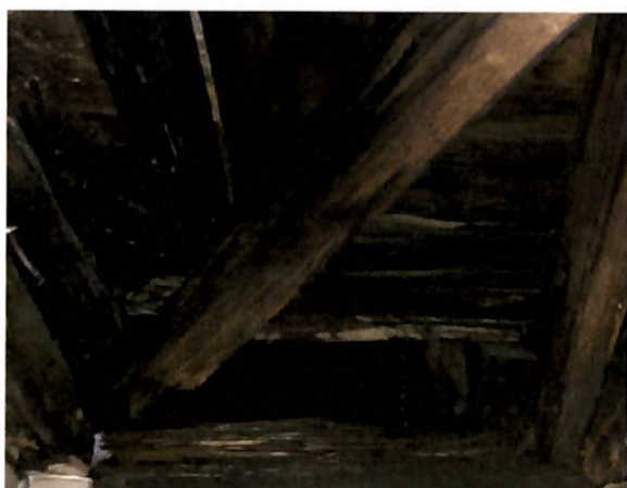
FIGURE 71 Deteriorated roof framing. Structura, Inc., 2019.
