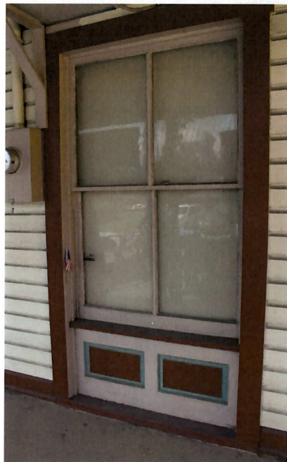
FIGURE 16 Two-over-two wood-sash double hung windows above a solid wood panel with two raised panels.
