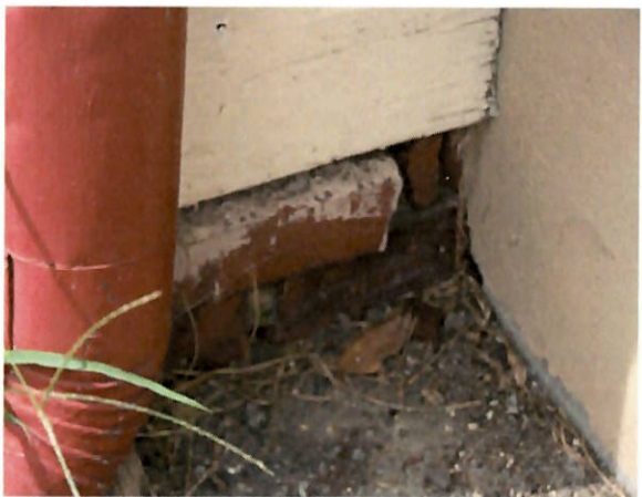
FIGURE 30 Detail, brick foundation, east elevation.
