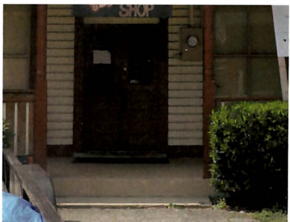
FIGURE 38 Painted concrete porch and step.
