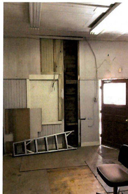
FIGURE 87 Interior, various layers of wall cladding materials revealed during exploratory demolition.
