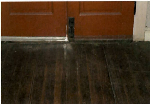
FIGURE 83 Interior, wood flooring at original construction.
