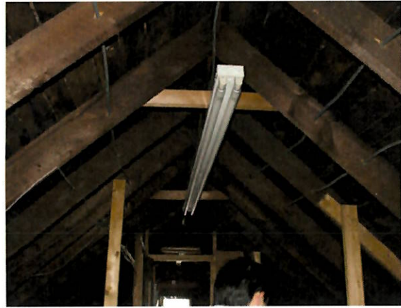
FIGURE 62 Gable roof framing.
