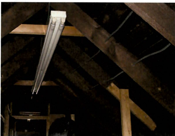
FIGURE 70 Sistered roof framing.
