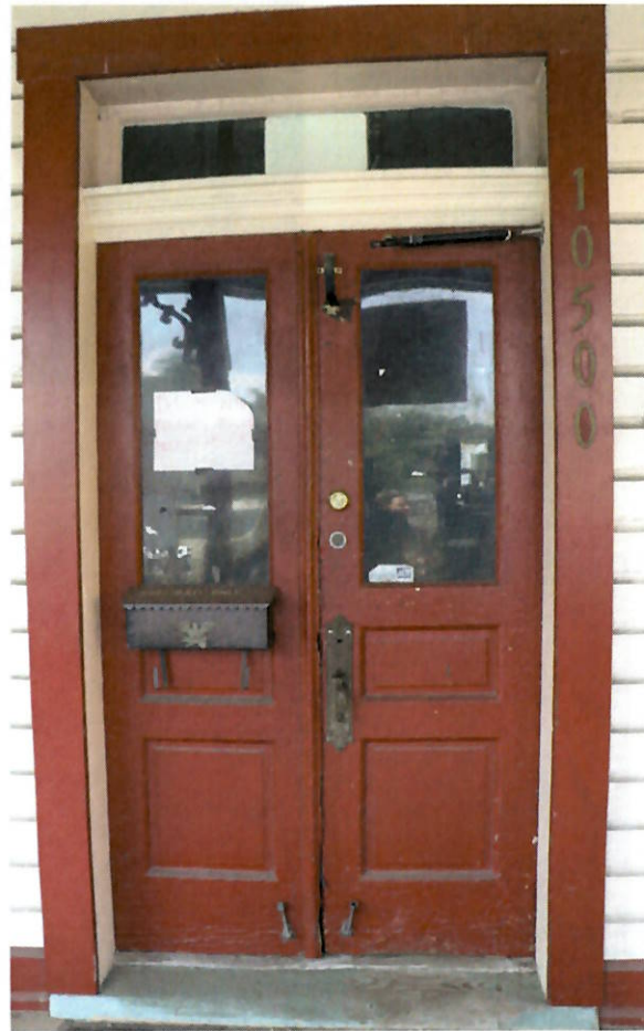
FIGURE 55 Double-leaf doors with two raised wood panels.
