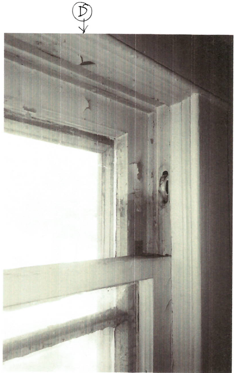
DETERIORATED WOOD WINDOW IN DINING RM.
