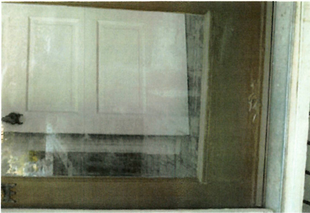
Side door - evident rot bottom panel
