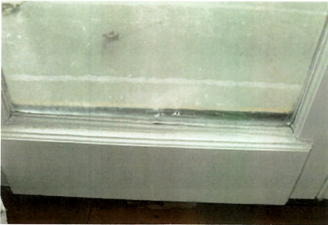
Balcony doors - buttressed/repared bottom panels - inside view
