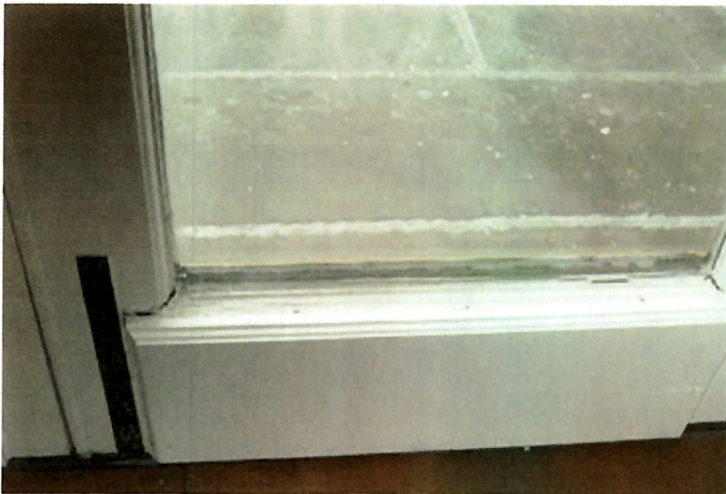
Balcony doors - buttressed/repared bottom panel - inside view
