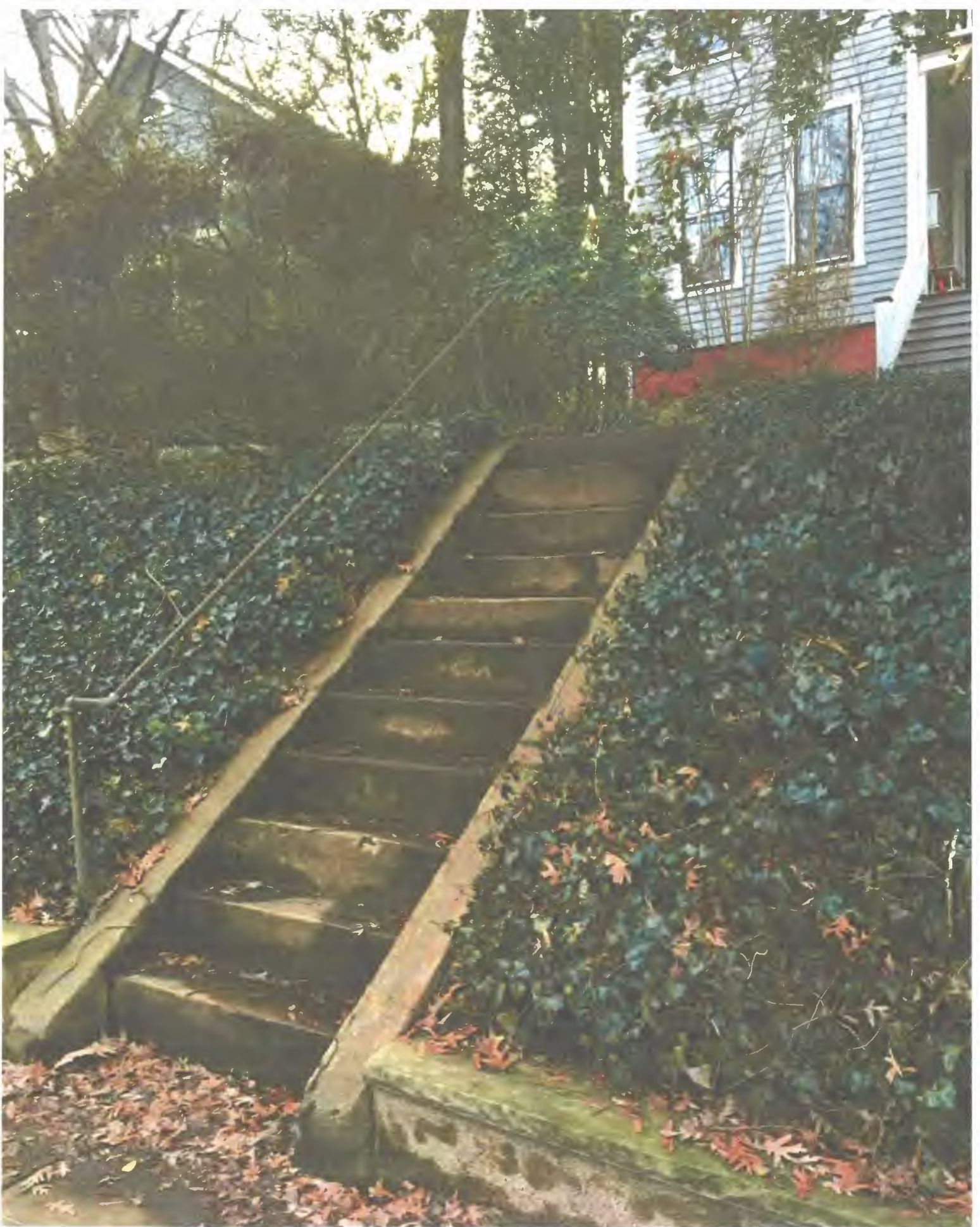
CURRENT FRONT STEPS (NOT UP TO CODE)
