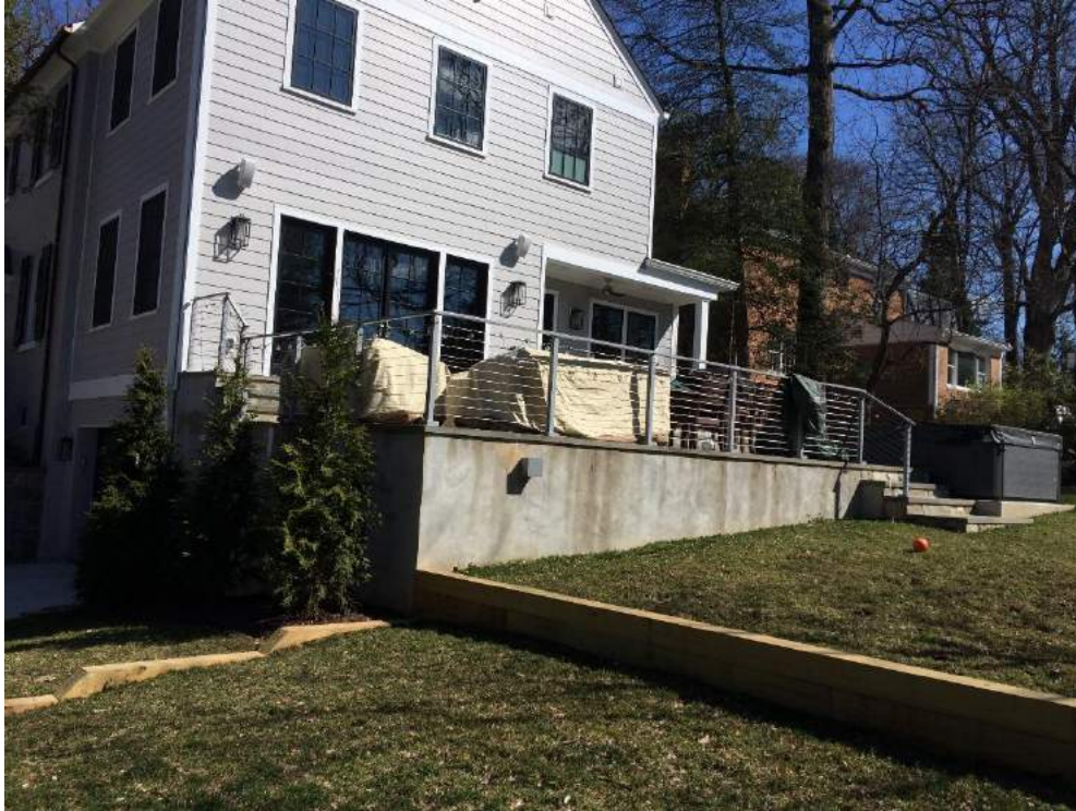
Fig. 6: As-built patio with high-tension cable railing.
