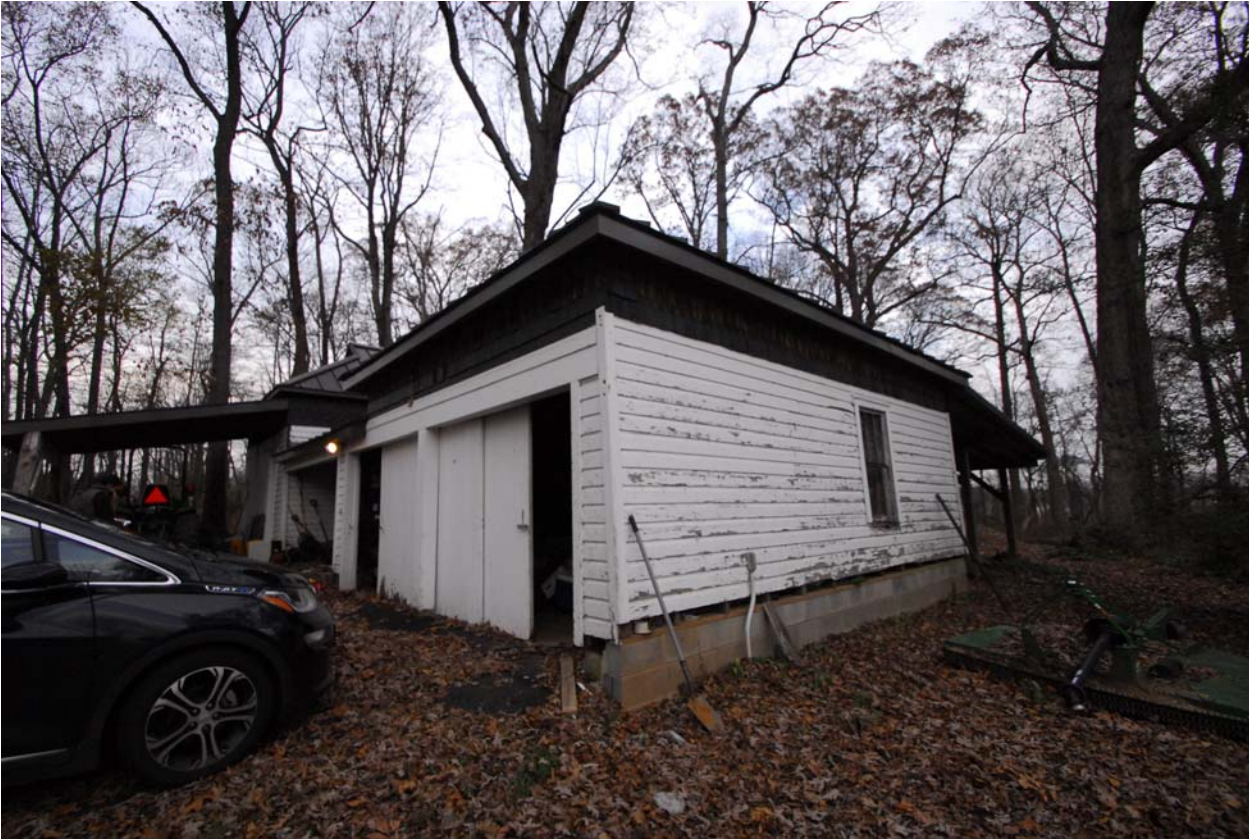
Figure 3. South facade and corner of structure.
