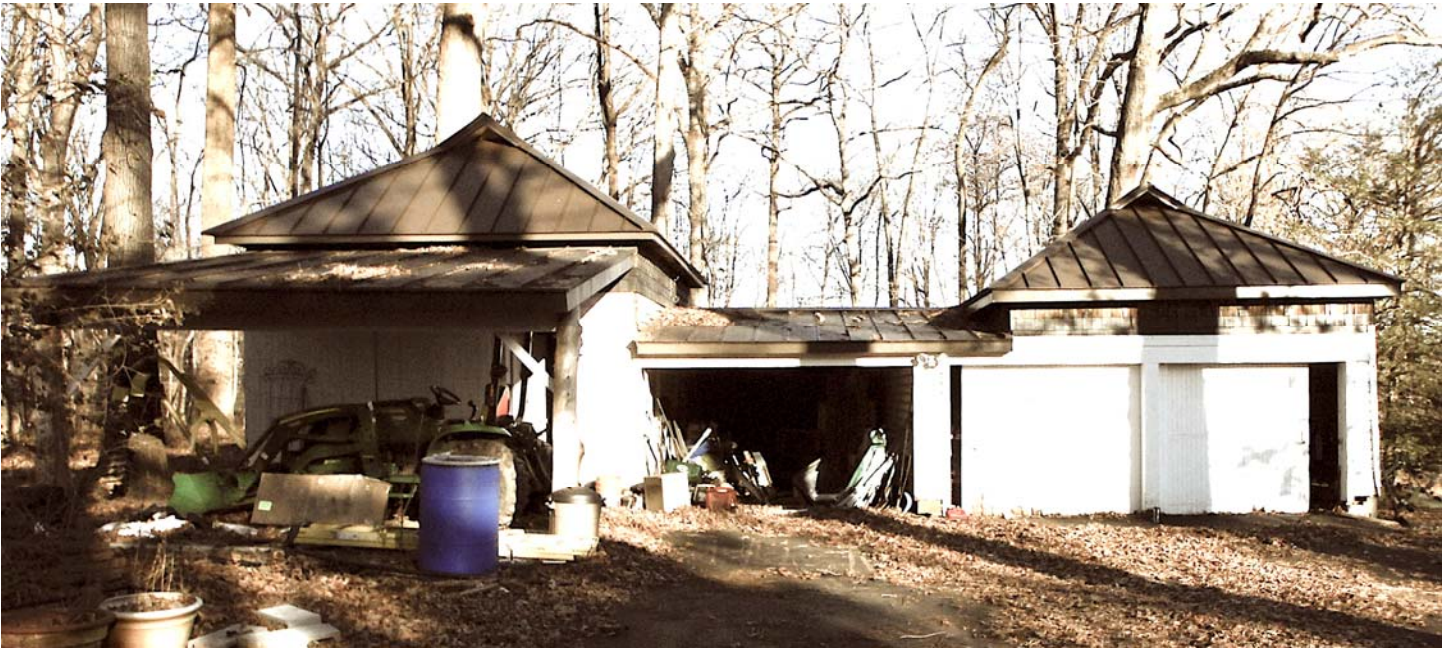
Figure 1. Front (west) facade showing garage and hyphen structure to be renovated.
