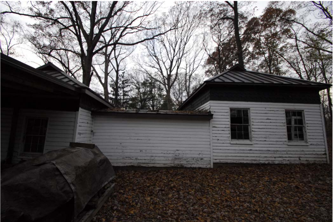
Figure 4. East facade showing hyphen and northern pavilion (to be renovated).
