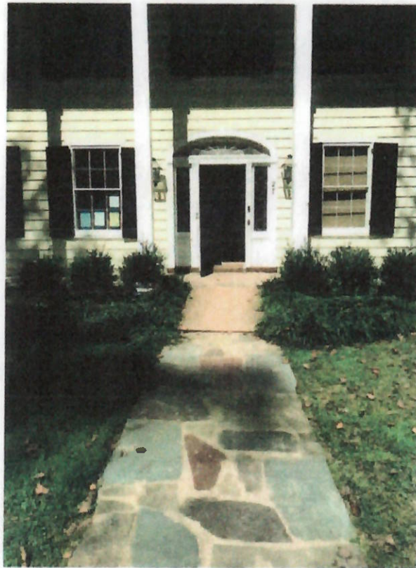
Existing front walk of flagstone on concrete. S view
