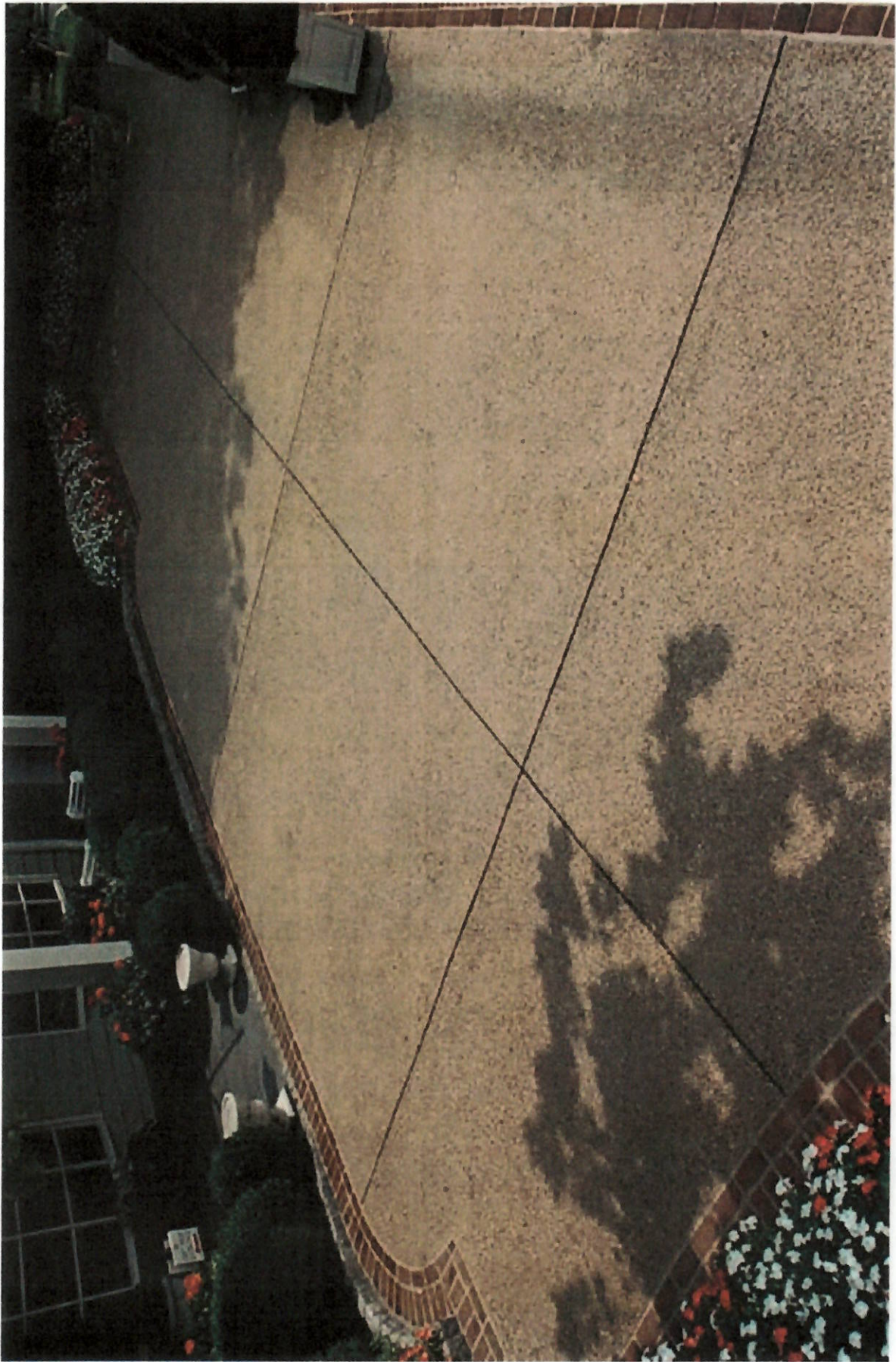
Exposed Aggregate driveway with Brick Edging
