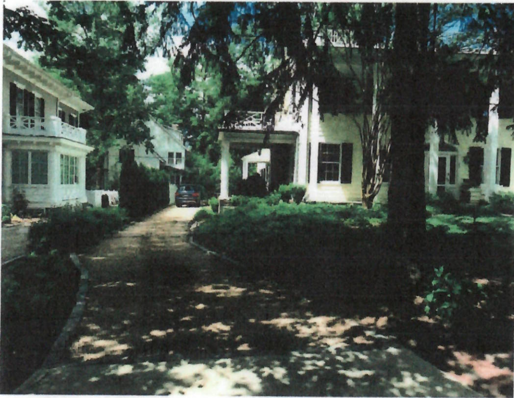
Existing gravel driveway edged with cobblestone, SW view
