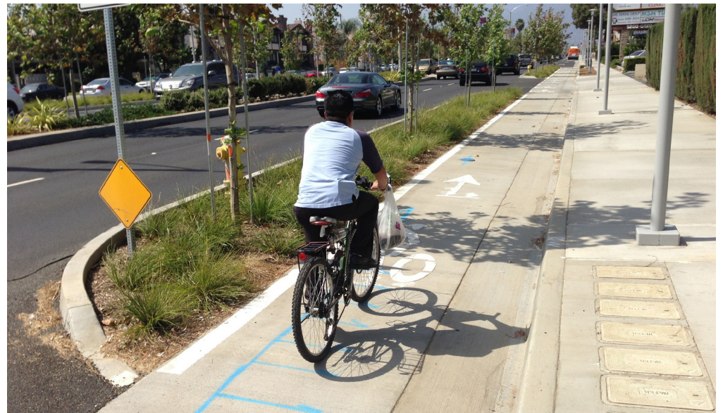
Separated bike lanes, street trees and planting strips provide additional buffering for pedestrians. Source: NACTO (above), Joe Linton/Streetsblog L.A. (below)
