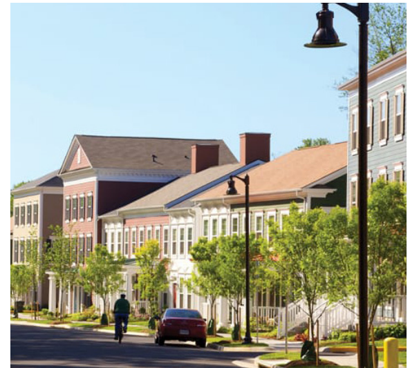
This development in Fairfax, VA knits the design of new flats, townhouses and duplexes into the surrounding community. Source: Torti Gallas + Partners
