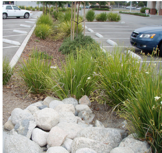
Stormwater management and planting in and along parking lots can reduce impervious surface and create more attractive sidewalks. Source: lacreek.wordpress.com
