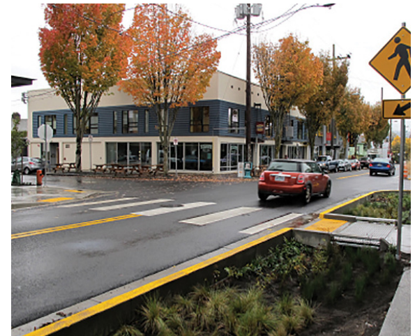
New development can reinforce the character of Industrial Mixed-Use Streets and provide enhanced streetscape, crossings and stormwater management. Source: NACTO
