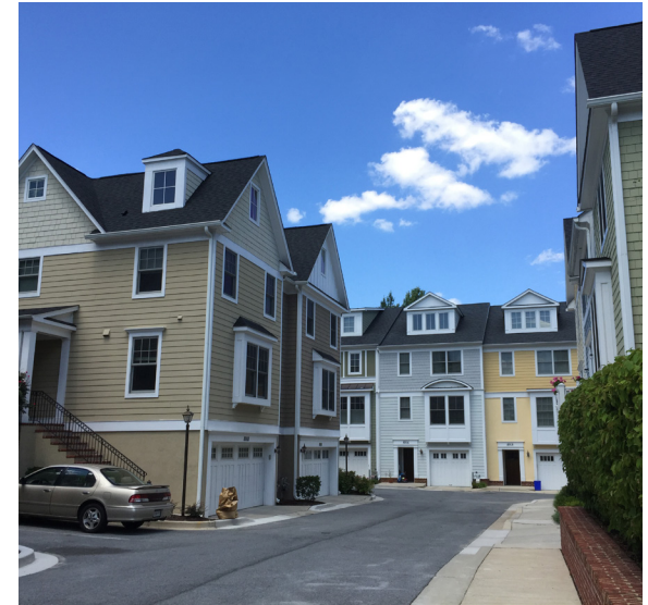
Townhome garages accessed from internal alleys to allow entries and frontage on the primary sidewalks. Source: M-NCPPC
