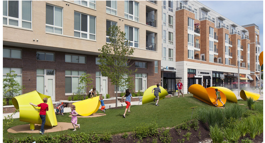
Ground-floor residential entries and retail open onto this public space creating an activated outdoor area. Source: Design Collective
