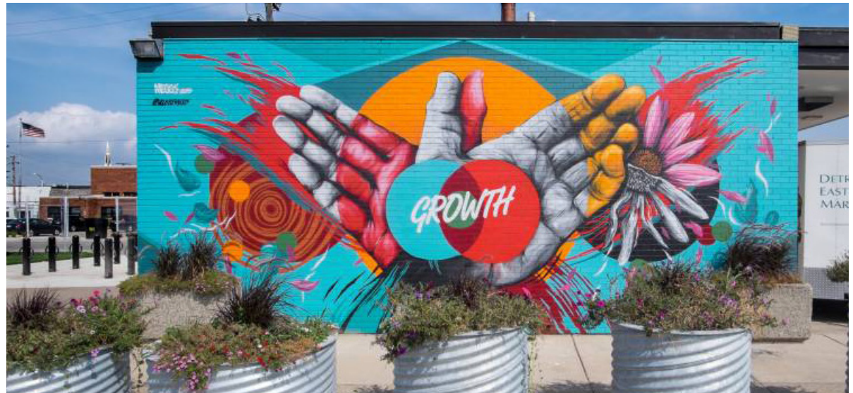
Facade improvements and mural art can be low-cost solutions to dramatically enhance the identity of the industrial area. Source: Jesse Cory
