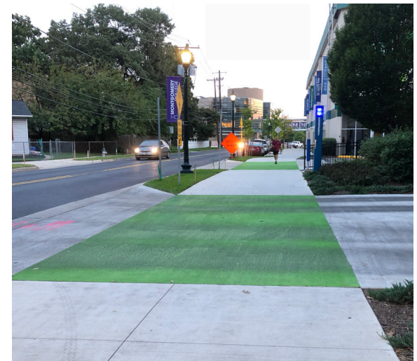
On streets like Brookville Road with frequent driveways, paint can help to indicate the continuous sidewalk Pedestrian Through Zone and encourage drivers to yield. Source: M-NCPPC
