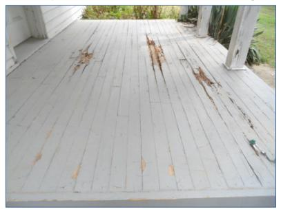
on the top surface will lose its adhesion and peel away due to the high moisture content within the lumber.
