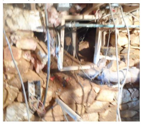
This area of the foundation is compromising the structural support for the building and should be addressed to prohibit further damage.
