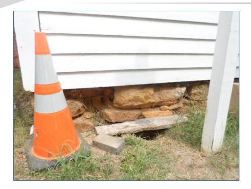
At the northeast corner of the cellar daylight entering between the wood structure and the stone foundation is due to missing stonework which should be repaired for preserving the structure. See recommendations below.
