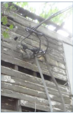
The electrical panel mounted inside the structure is exposed to weather with evidence of water on the panel (*see inset photo*). The circuit breakers are exposed with no blank plates over empty breaker slots. The panel and breakers are not intended for an exterior application, which is essentially the case given the weather exposure, and poses serious risks and creates a hazardous condition.
