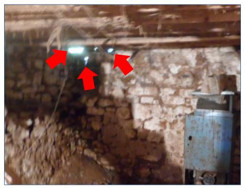
Some repointing work appears to have been performed along the east wall of the foundation in the cellar; however, the appearance of the mortar used for repointing indicates a high content of portland cement which further damages stone foundations, especially below grade.
