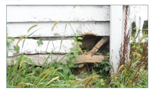
**Deferred Maintenance Condition – Front Porch Floor:** The front porch floor is showing signs of rot and deterioration. Although the floor boards were painted at some point in time, the wood appears to have been still absorbing and retaining moisture – probably due to their orientation perpendicular to the floor slope. Additionally, if the other three surfaces of each board are not primed or treated to resist absorption, the paint
