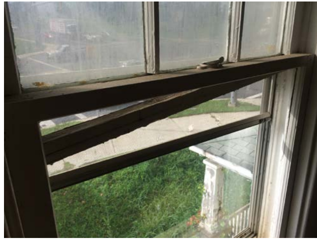
Figs. 2 & 3: Deteriorated Second-Floor Window, Southeast Elevation
