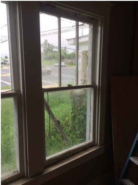
Figs. 2 & 3: Deteriorated First-Floor Window, Southeast Elevation
