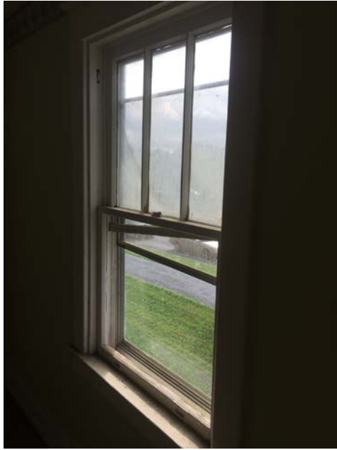
Figs. 2 & 3: Deteriorated Second-Floor Window, Southeast Elevation
