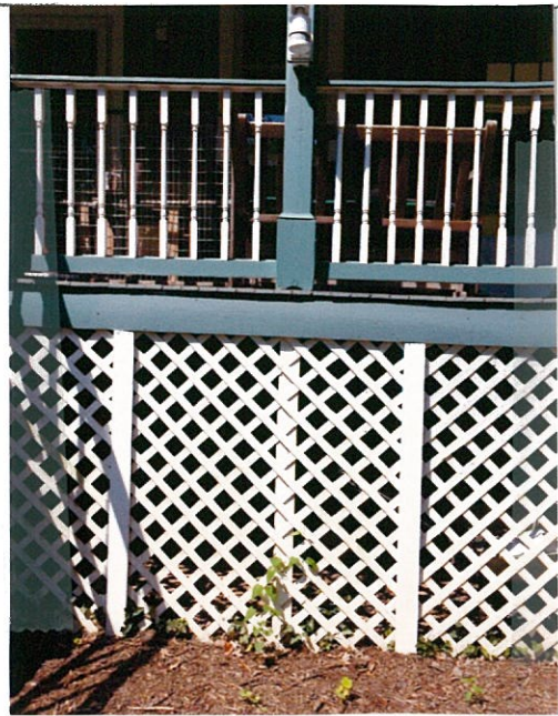
Rear Porch Columns are stacked over foundation posts but are not trimmed flush w/beam and posts
