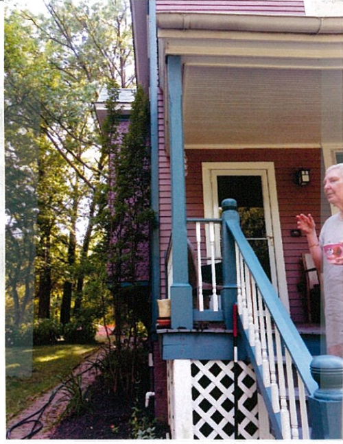
Rear Porch w/4 1/2" chamfered columns w/ plinth block
