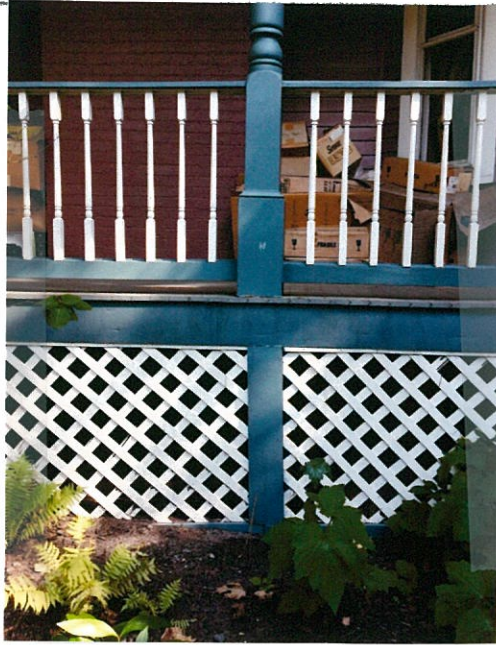
Front Porch Columns stack directly over foundation posts and are trimmed flush w/beam and posts
