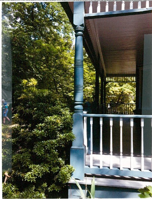
Front Porch w/5 1/2" turned columns, pedestal base, plinth block & entablature w/beveled cap
