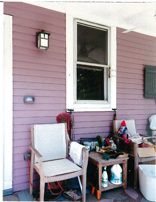
Kitchen window onto Rear Porch w/truncated head casing
