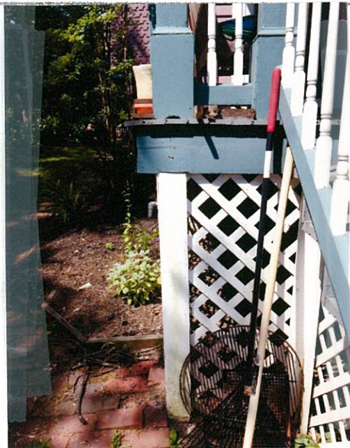
Rear Porch Columns are offset over foundation and trim is not flush w/beam and columns @ corner
