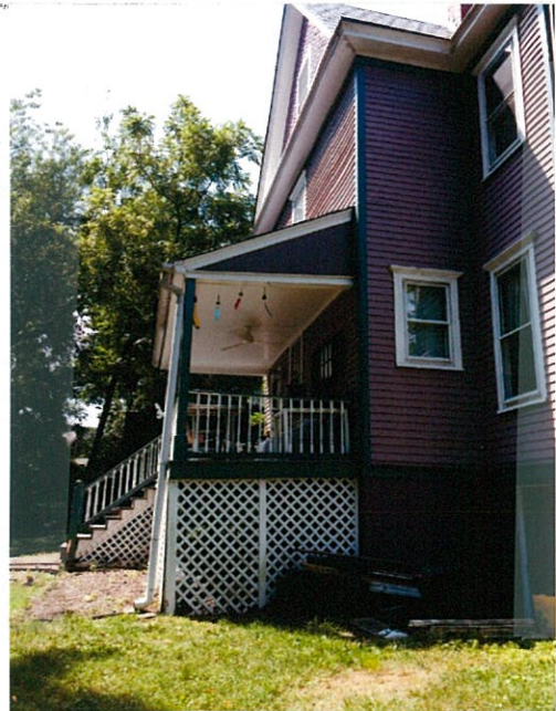
Rear Porch steep floor slope
