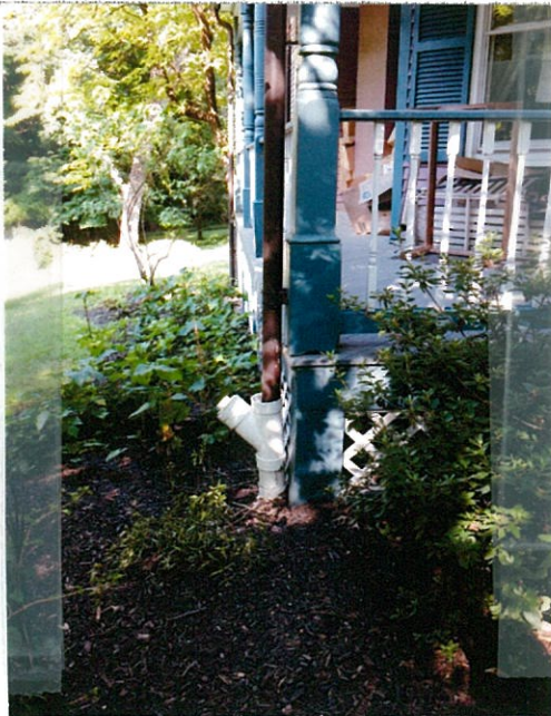
Front Porch Columns stack directly over foundation and trim is flush w/beam
