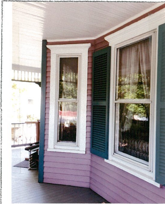
Living Room Windows onto Front Porch w/full head casing
