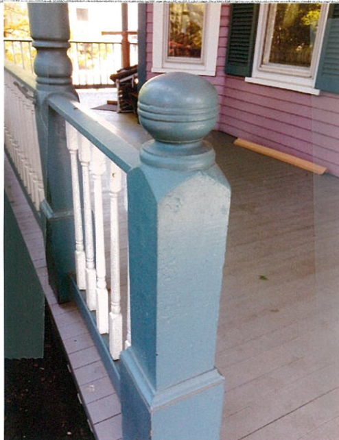
Front Porch Knewel w/shallow bevel @ final & plinth block
