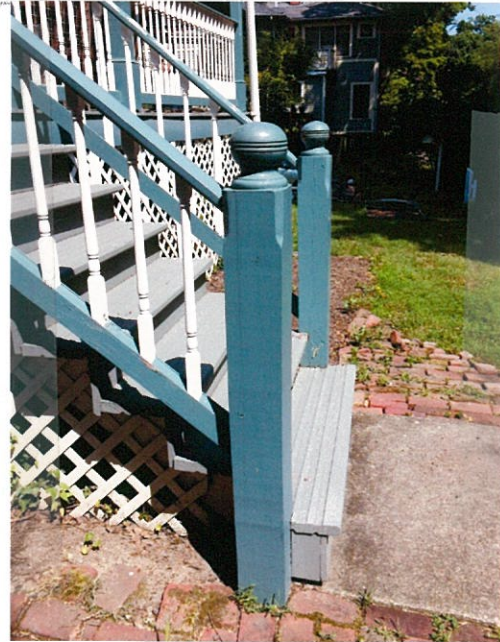
Rear Porch Knewel w/longer beveled corners and no plinth block
