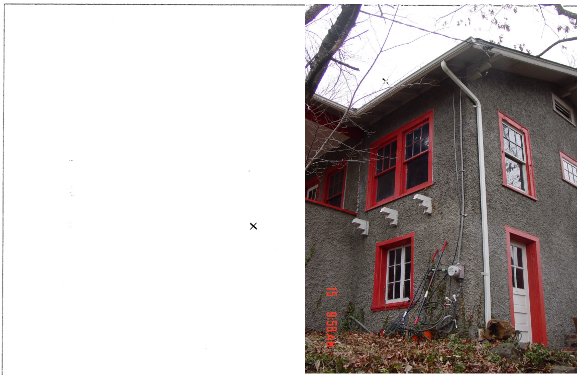
Detail: 7015 Sycamore Ave. Right hand front elevation cellar casement and bracket detail
