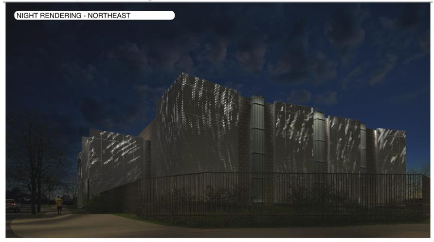
In lieu of fenestration, the use of backlit perforated Trespa laminate panels creates a visually light scrim over the concrete shell. A CNC-routed pattern depicting waves of energy is applied to the panels, which has a subtle daytime quality and becomes an illuminated nighttime feature facing the streets. Vertical channel glass 'lanterns' between the bays animate the building with light and introduces glass to the project material pallet without using traditional windows.
