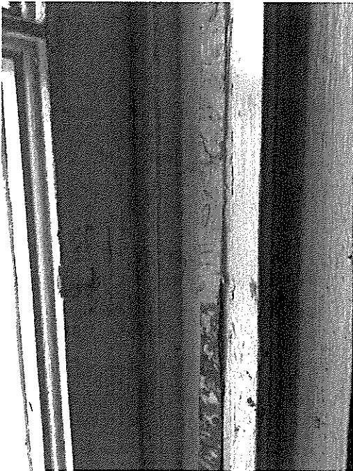
Photo C. 'Strap pulley' window with intact strap and damaged stile
