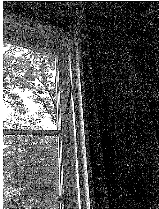
Photo D. 'Strap pulley' window with detached strap
