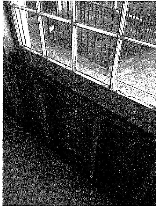
Photo H. Twelve-over-twelve window, replacement bottom rail
