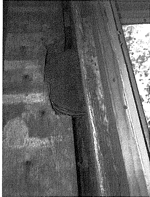
Photo B. Detail of 'strap pulley' cassette, set into four by four stud
