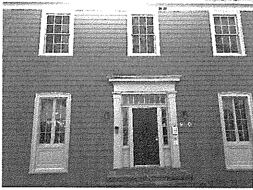
Photo A. Exterior, six-over-six 'strap pulley' cassette sash windows (top) and casement windows (bottom)
