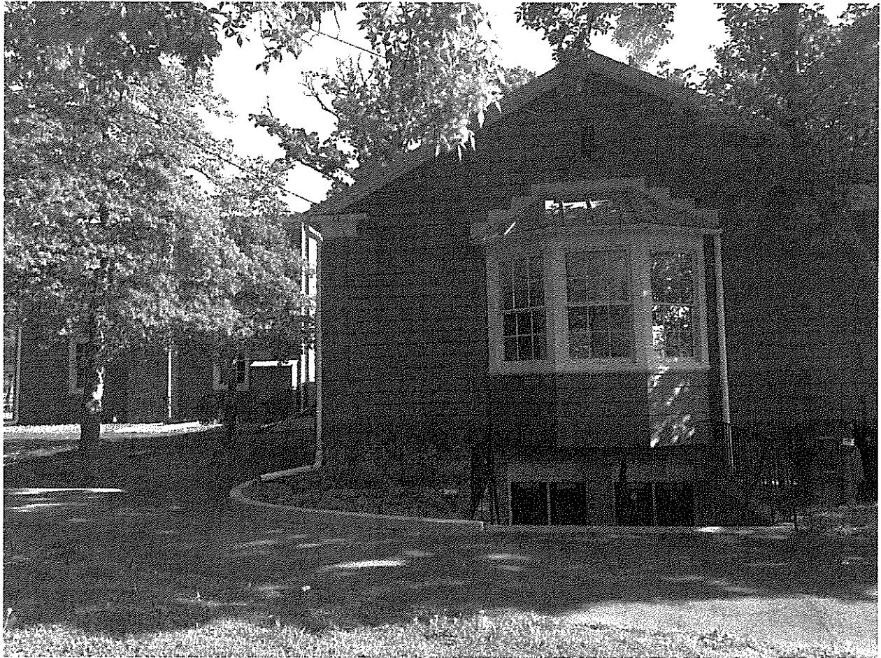
Areaway providing access to library wing basement.
