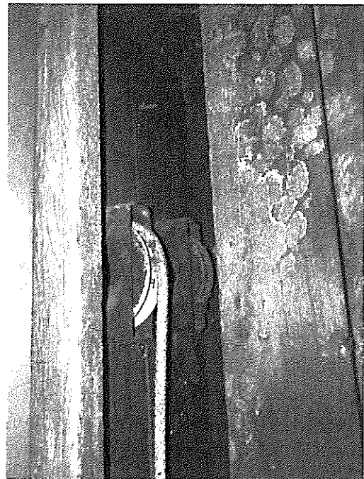
Photo J. Detail, pulleys from double-hung window
