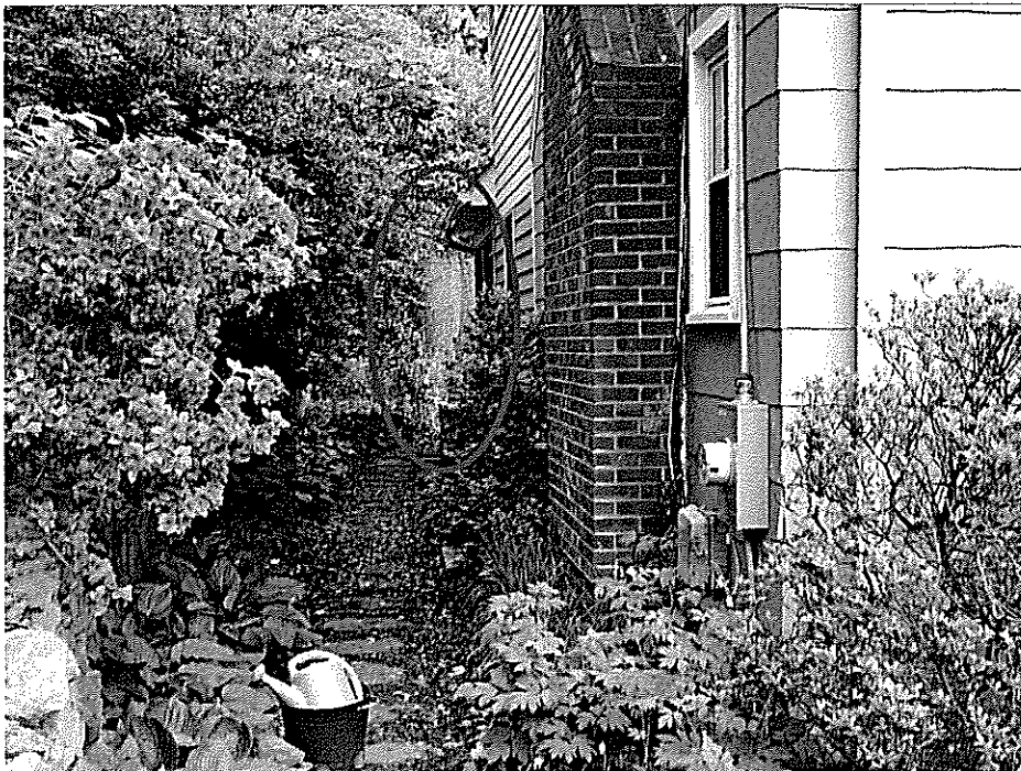
Figure 3: Closer view showing right side of house with stumps minimally visible.
