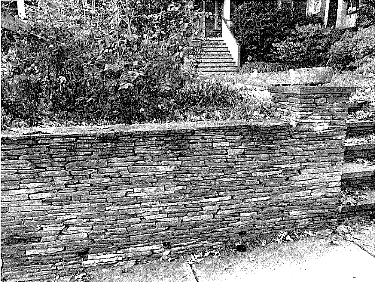
Figure 2: 7112 Holly Ave. retaining wall in the materials and design proposed for the subject property (Image provided by applicant).
