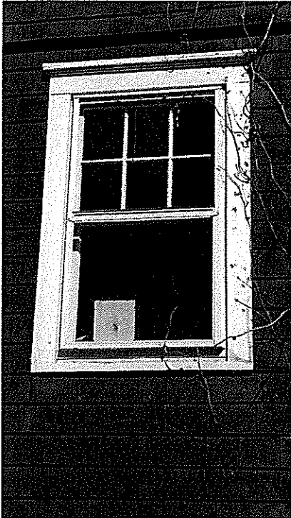
Existing windows in main house are single glazed, wood frame and sash with storm windows
