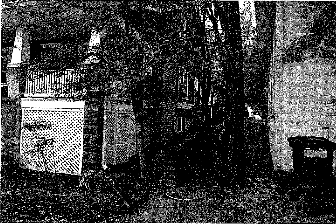
View from sidewalk on Westmoreland of right side, existing windows will be replaced in existing openings.
