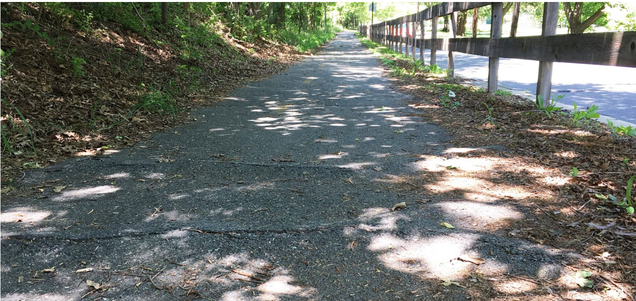
Pavement cracking is common on sidepaths
