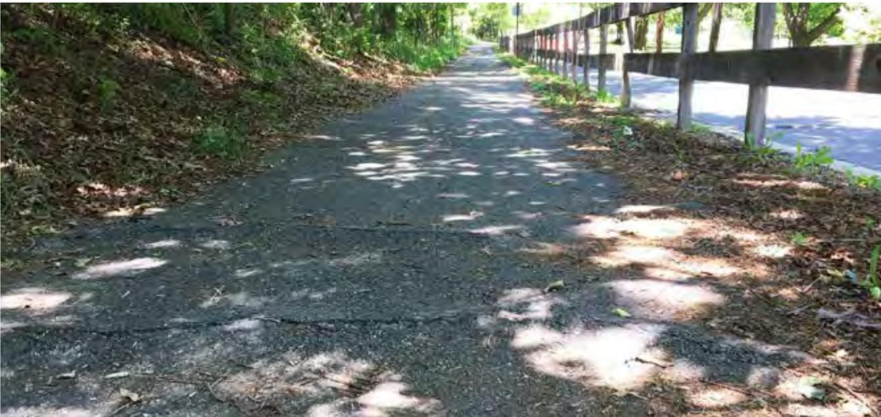
*Pavement cracking is common on sidepaths*
