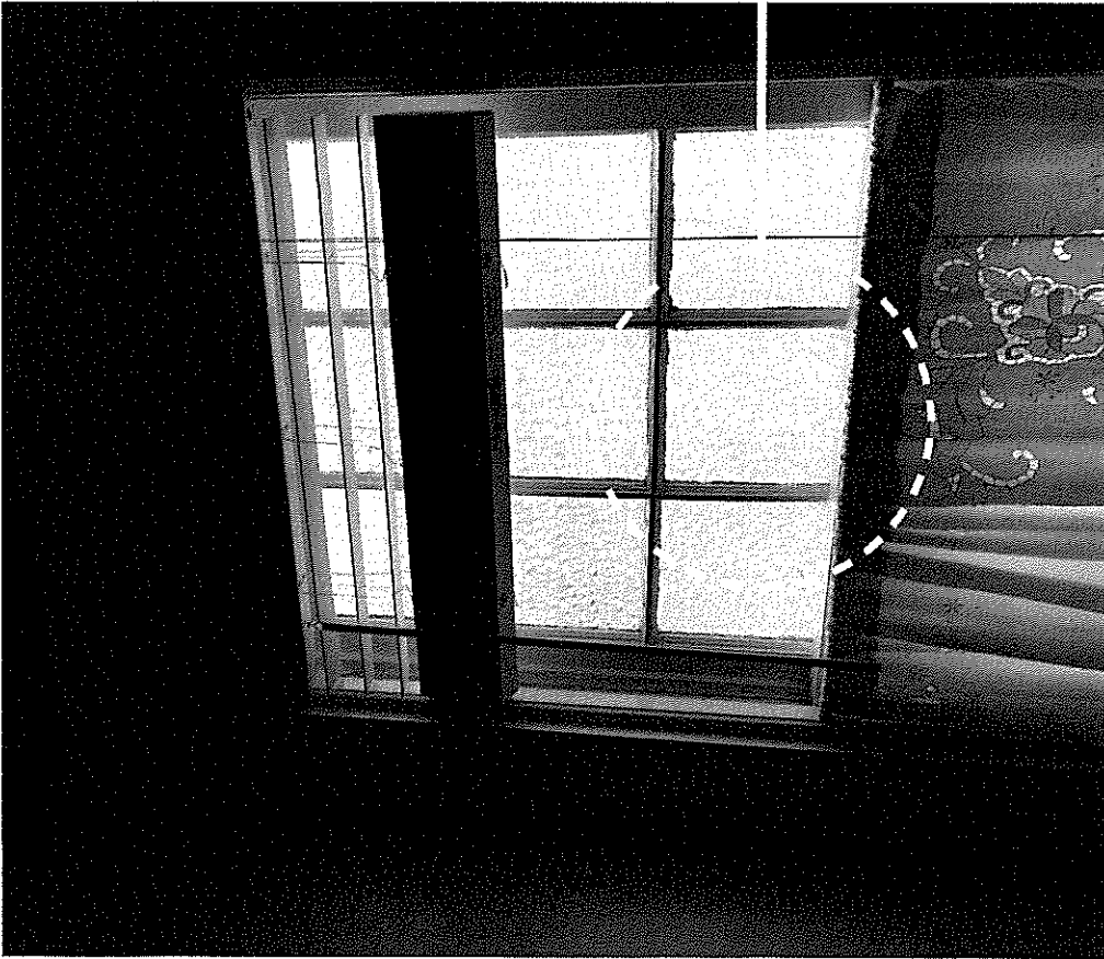
WINDOW '1': HISTORIC WINDOW (VIEW FROM INTERIOR) PROPOSED WORK: RE-GLAZE EXISTING WINDOW AND REPLACE WITH NEW SINGLE PANE LAMINATED OBSCURED GLASS; NO OTHER ALTERATION OF WINDOW IS PROPOSED.
