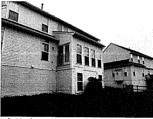
Left side of rear of home (showing neighbor at 18625)
