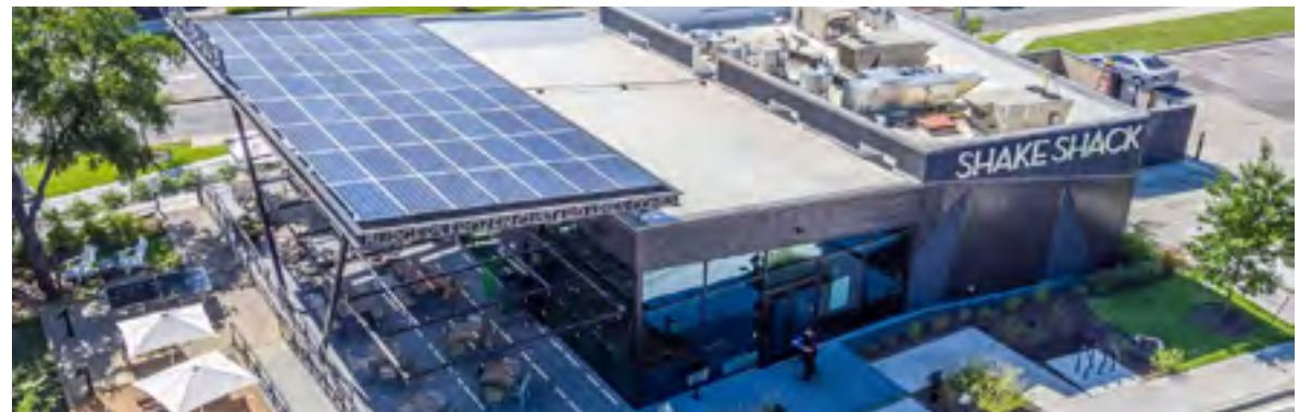
This building is fitted with solar panels and a cool roof to reduce energy costs. Both sustainable design elements and site design led to a LEED rating for the building.
