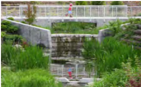
Through weirs, natural channels and terraces, this daylight stream transforms from a buried pipe to a thriving habitat for plants, animals and people.
