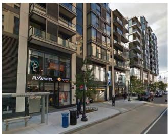
This parking entrance is designed to blend with the ground floor retail design, and has a limited driveway width to reduce interruption along the sidewalk.
