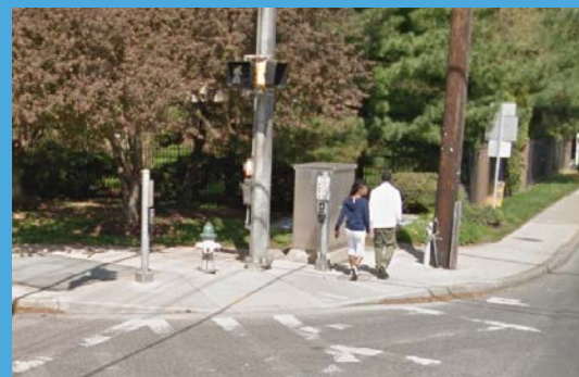
Existing curb ramps at northwest corner of Georgia Avenue and Forest Glen Road (Recommendation 32)
