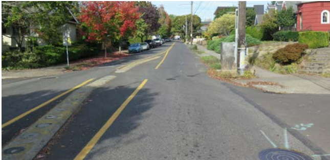
Off-set intersection bicyclist left turn median diverter
