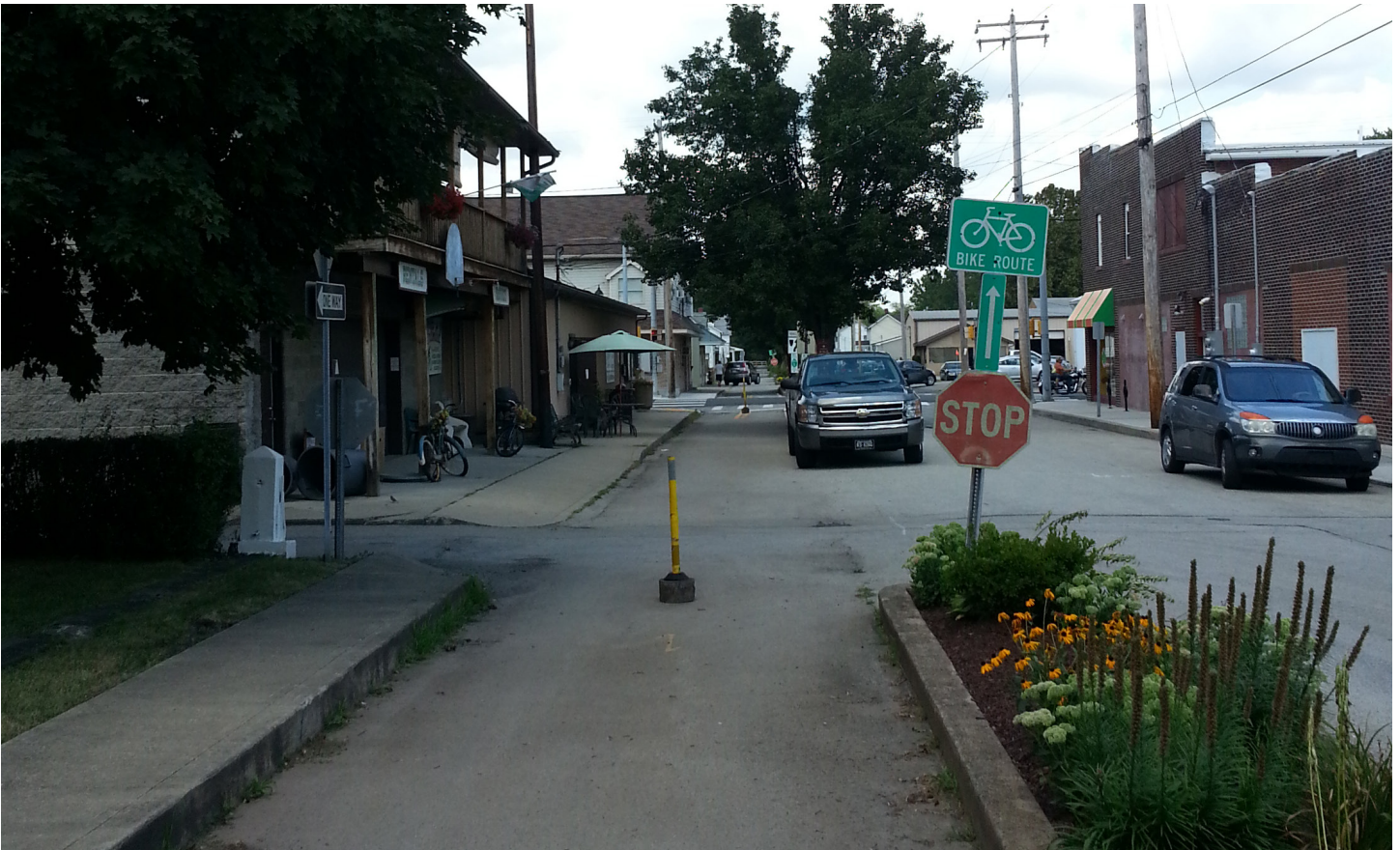
Raised medians provide separation from traffic for these bike lanes. Source: Jeremy Chrzan
