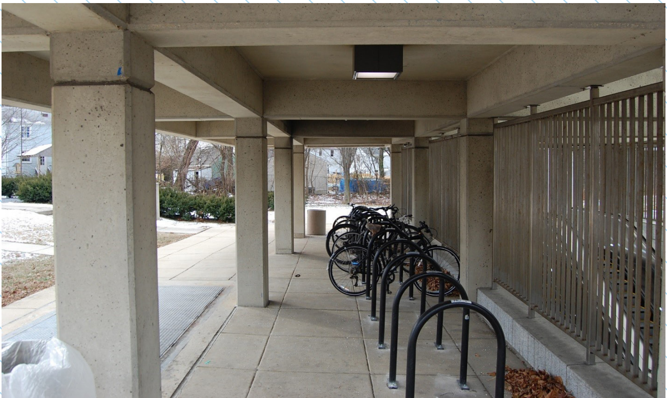
Covered short-term bicycle racks at the Glenmont Metrorail station
