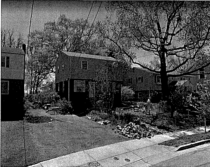
Pre-renovation/addition, East view
