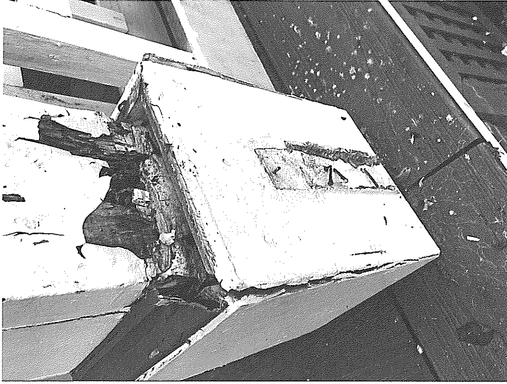
FRONT PORCH POST BASE (TO BE REPAIRED/ REPLACED TO MATCH)
