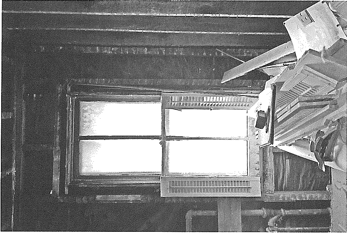
SECOND FLOOR WINDOW (FIRE DAMAGED/TO BE REPLACED)
