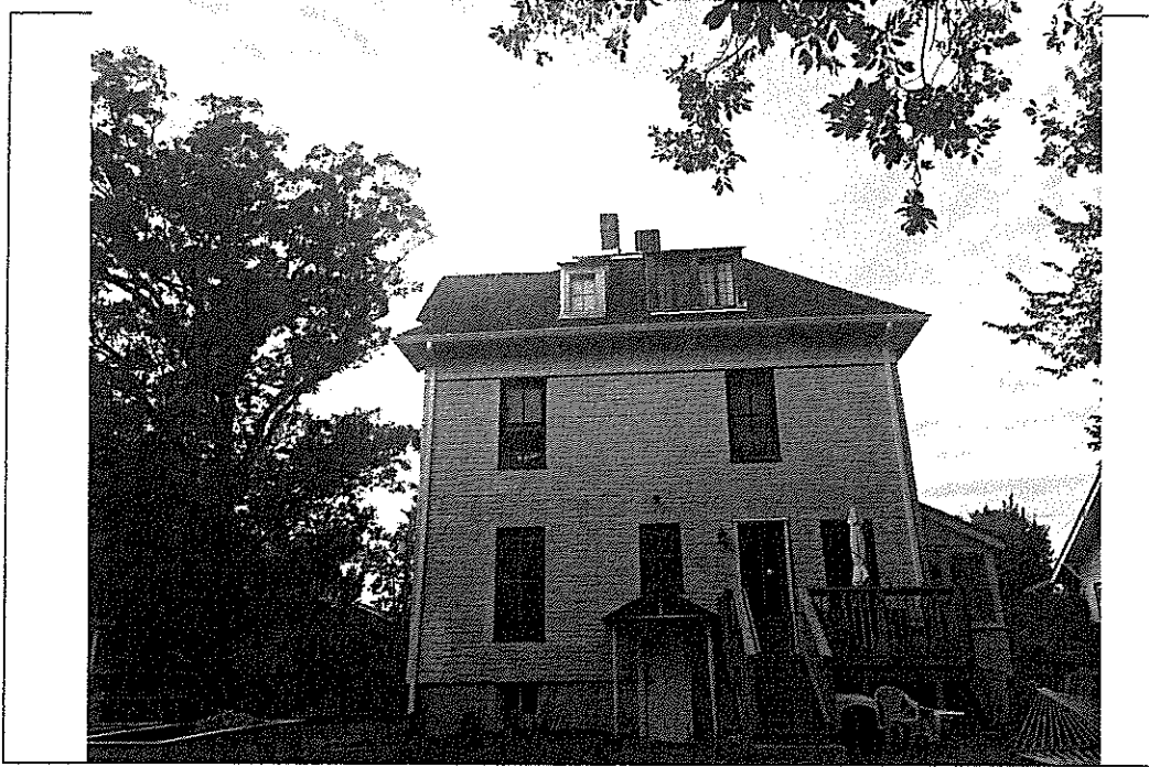
Detail: Rear facade
