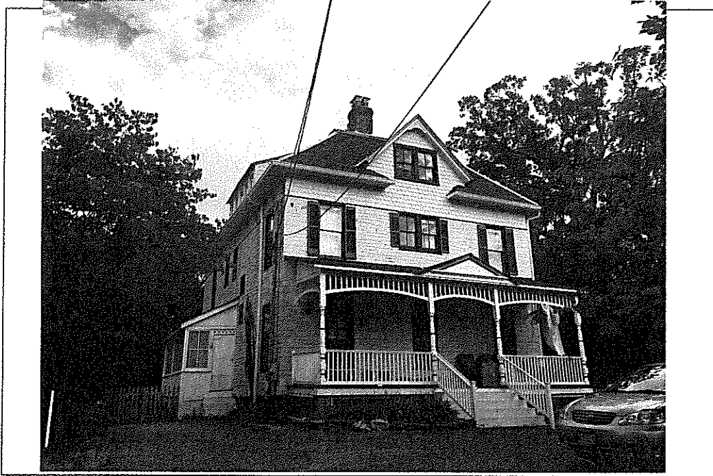
Detail: Front facade from street #2
