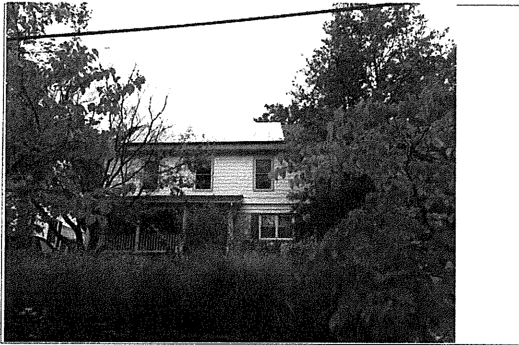
Detail: South rear-adjacent neighbor from public right of way 26 Columbia
