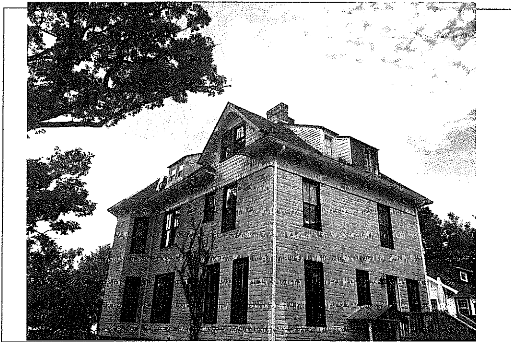
Detail: South (side) facade
