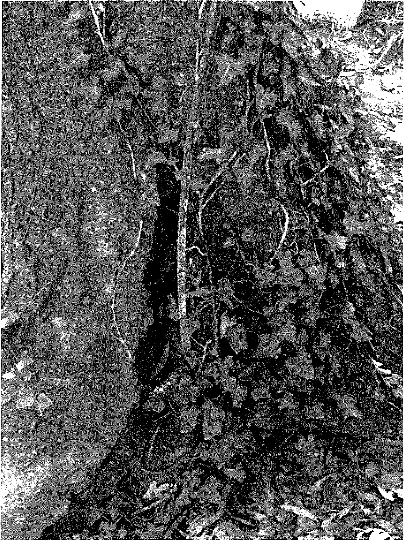
Tree base with rot damage
