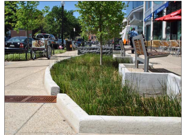
Planted area on sidewalk for stormwater management
