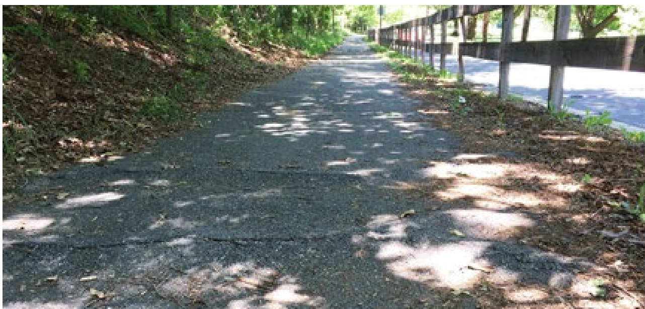
Pavement cracking is common on sidepaths
